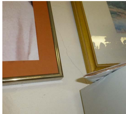
Figure 14: Cracking of plaster wall.
