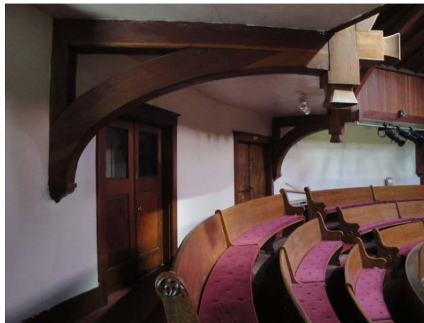
Detail of a knee bracket at the balcony.
