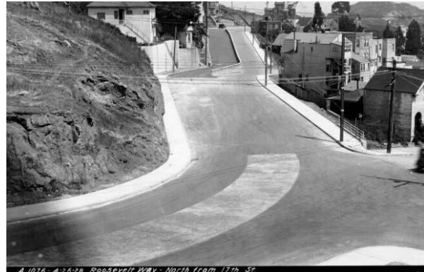
Figure 120 – 1928 view north on Roosevelt from Seventeenth showing utility poles and wire as well as new asphalt topped macadam paving. (San Francisco History Center, San Francisco Public Library. AAB-5165)
