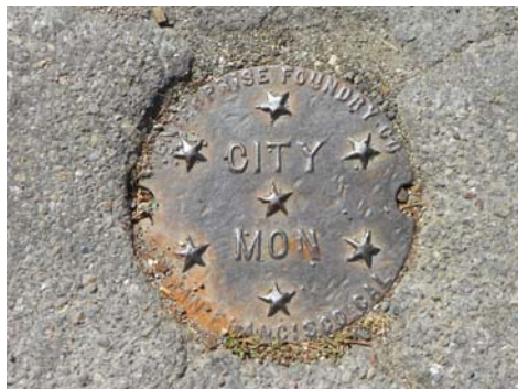
Figure 166 – Hand hole cover for a City Monument, end of Saturn Street, manufactured by Enterprise Foundry Company, date unknown. (Photo by M.R. Corbett, 23 July 2012)
