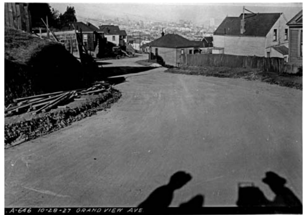
Figure 105 – 1927 view of macadam paving on Grand View. (Courtesy of Western Neighborhoods Project. Labeling consistent with Department of Public Works Photos.)
