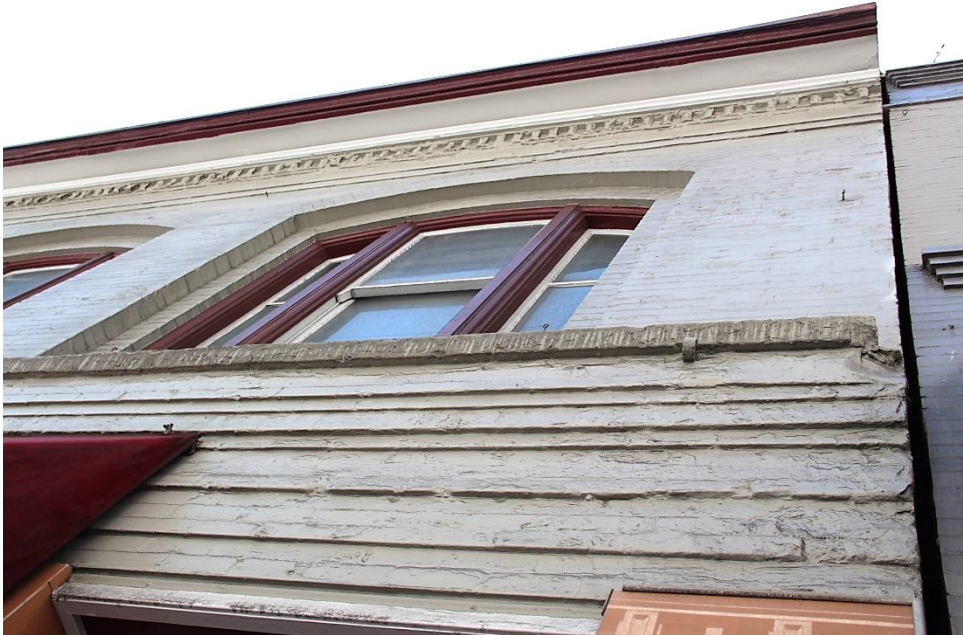
Detail of brick corbelling on the Second Street facade.
