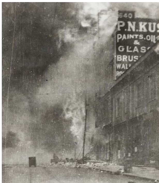
Fire burning at 640 and 644 Mission Street, a short distance west of New Montgomery Street (California Historical Society)
