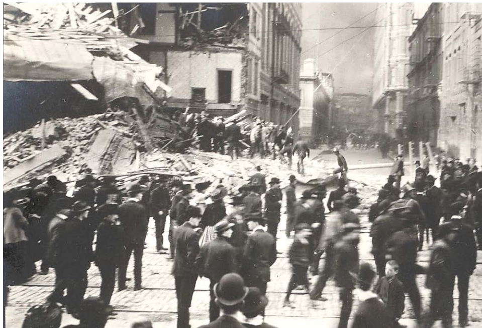
Rescue efforts at the Wilcox House, located only 75 feet north of the Bourdette Building at the southwest corner of Second and Jessie streets. The large building on the left beyond the wreckage is the Crossley Building. At right in the distance are the rear facades of the Grand Hotel and Palace Hotel. (Bancroft Library)
