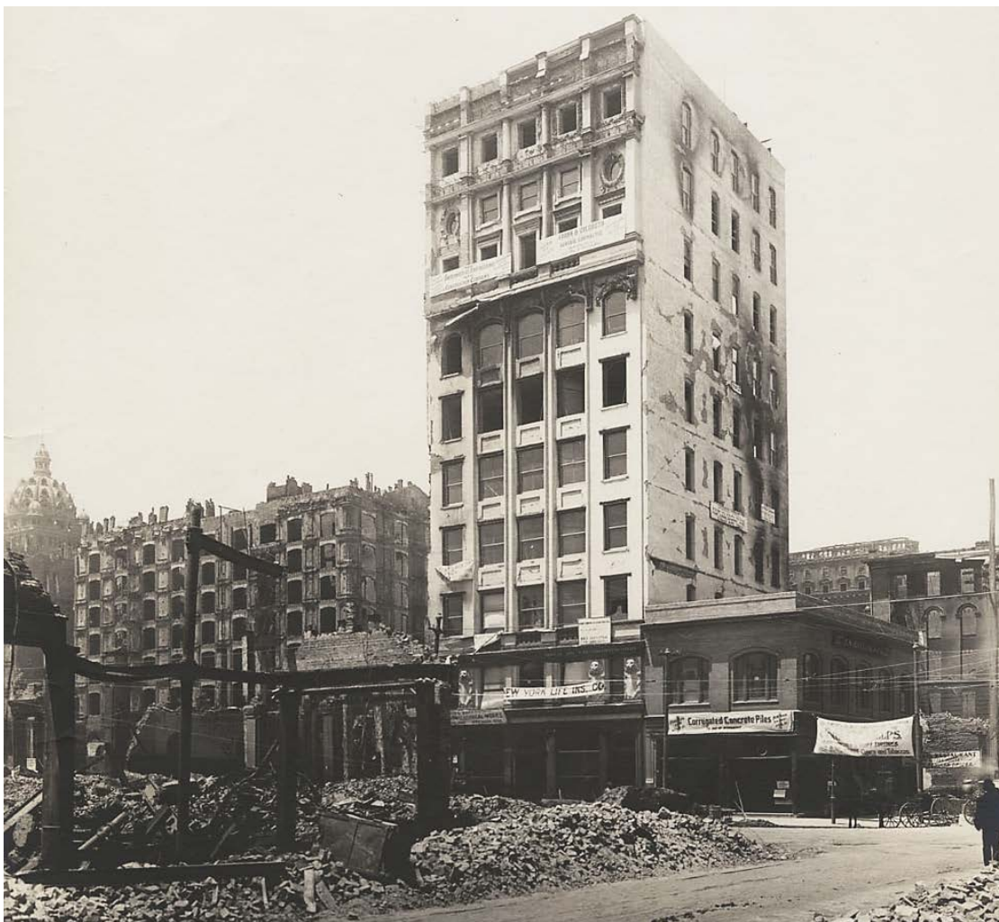
The Atlas and Bourdette buildings, May 15, 1906. Visible at left is the brick shell of the Palace Hotel and the dome of the Claus Spreckels Call Building. (Turnbull & Miller photo for the California Promotion Committee, California Historical Society collections)
