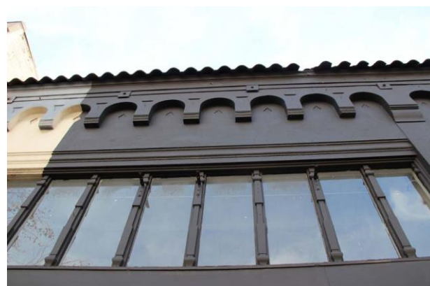
Figure 54. Detail of transom and frieze on primary façade. Source: Christopher VerPlanck
