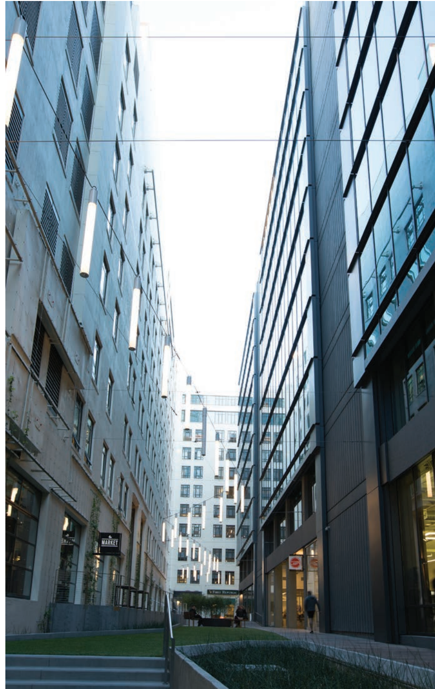
Stevenson Street, view looking east, after renovation (BCJ)
