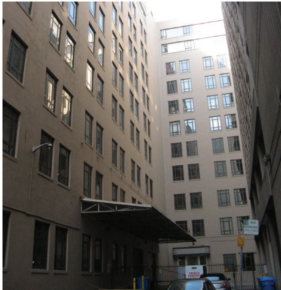
View of Stevenson Street from Tenth Street prior to the renovation
