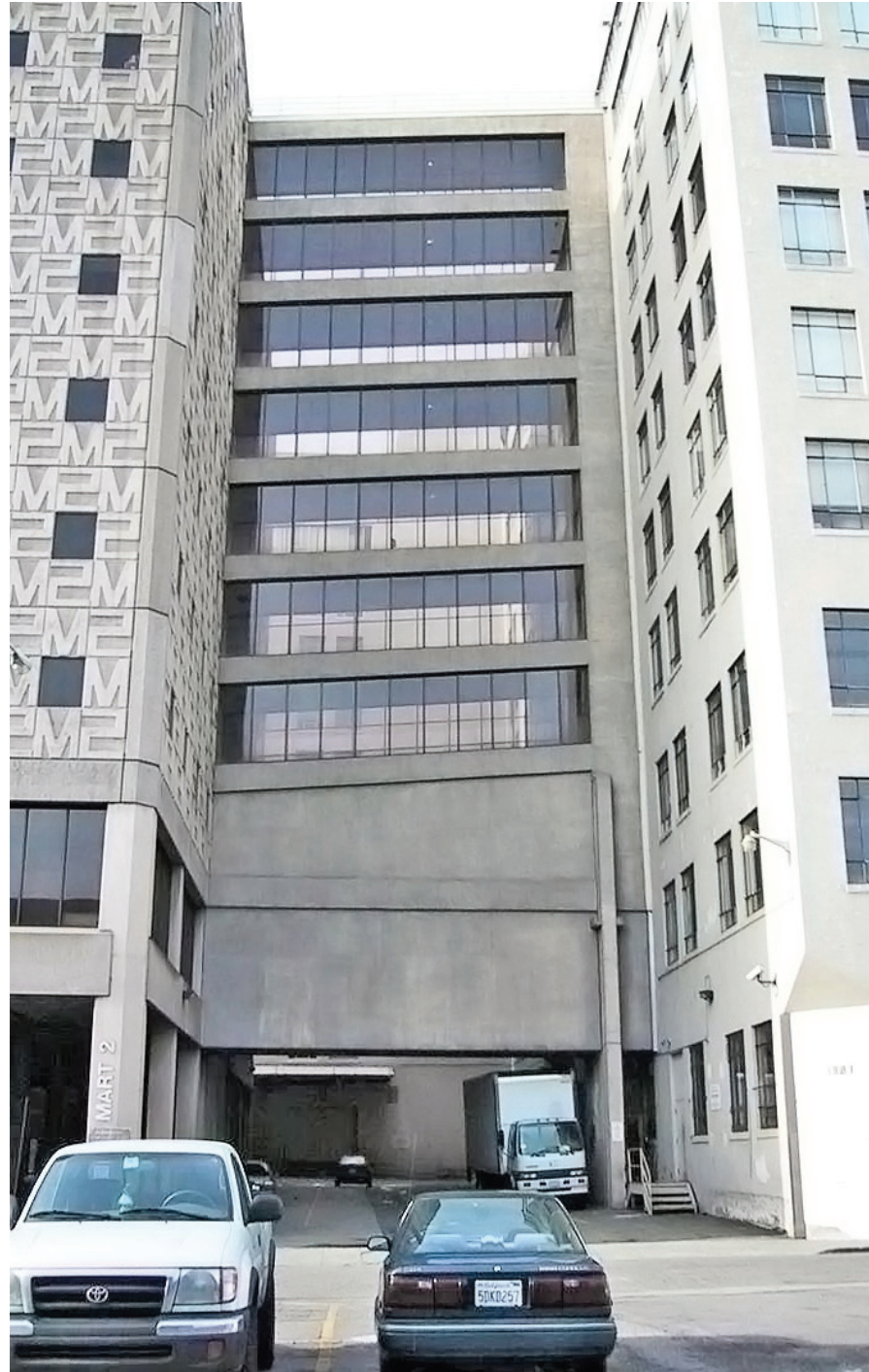
View looking north from Jessie Street of previous skybridge.
