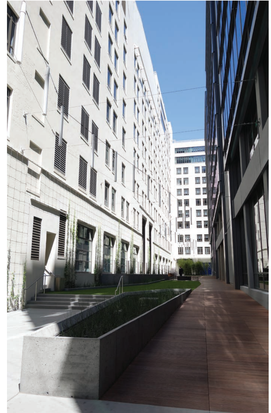
Stevenson Street, view looking east, after renovation (BCJ)
