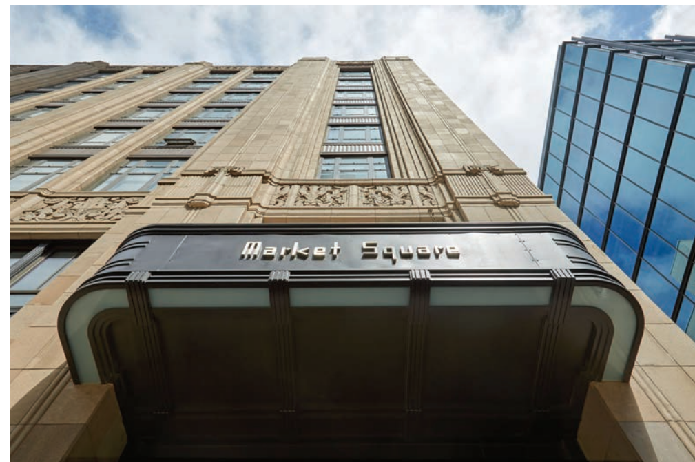
Historic canopy at Tenth Street (Bruce Damont)
