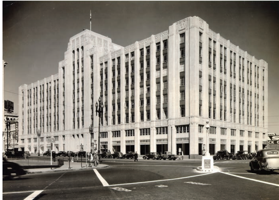
View southeast from corner of Tenth and Market Streets, 1937 (San Francisco Public Library Historical Photograph Collection (SFPL), #AAC-5020)
