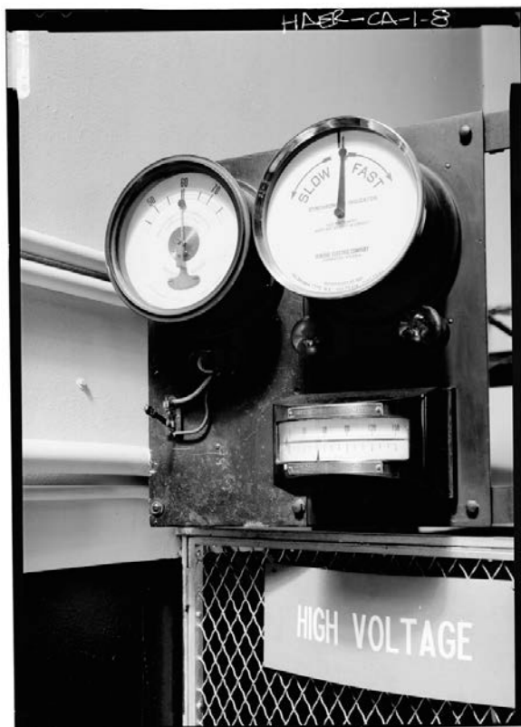
FIGURE 11 - Synchronizer indicator.
