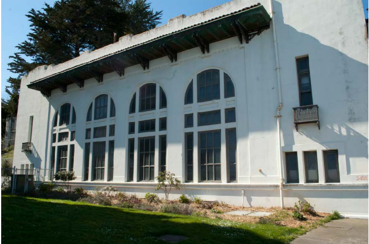
FIGURE 19 - Eastern side of Pump Station No. 2, showing windows to be replaced at the far right and left, and four sets of Bay windows (to remain) in the center.
