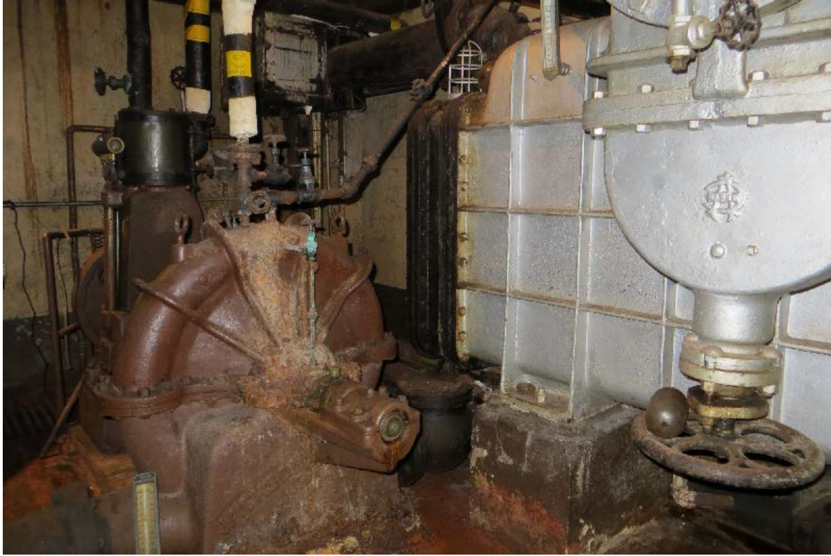
FIGURE 15 - Basement circuit pump (brown equipment at left) and condenser (silver equipment at right)
