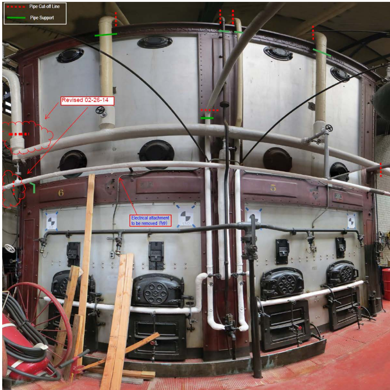
FIGURE 3 - Piping in front of a boiler (Boilers 5&6)
