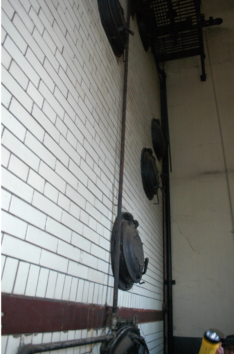
FIGURE 2 - Side of a boiler showing glazed tiles
