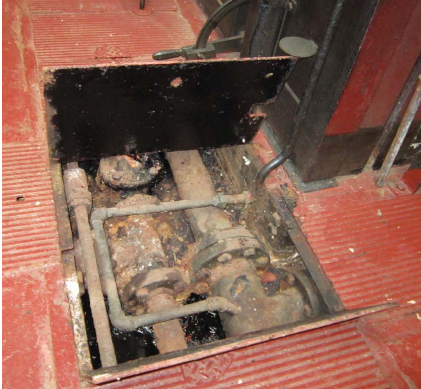
FIGURE 7 - Boiler trench with trench plates removed
