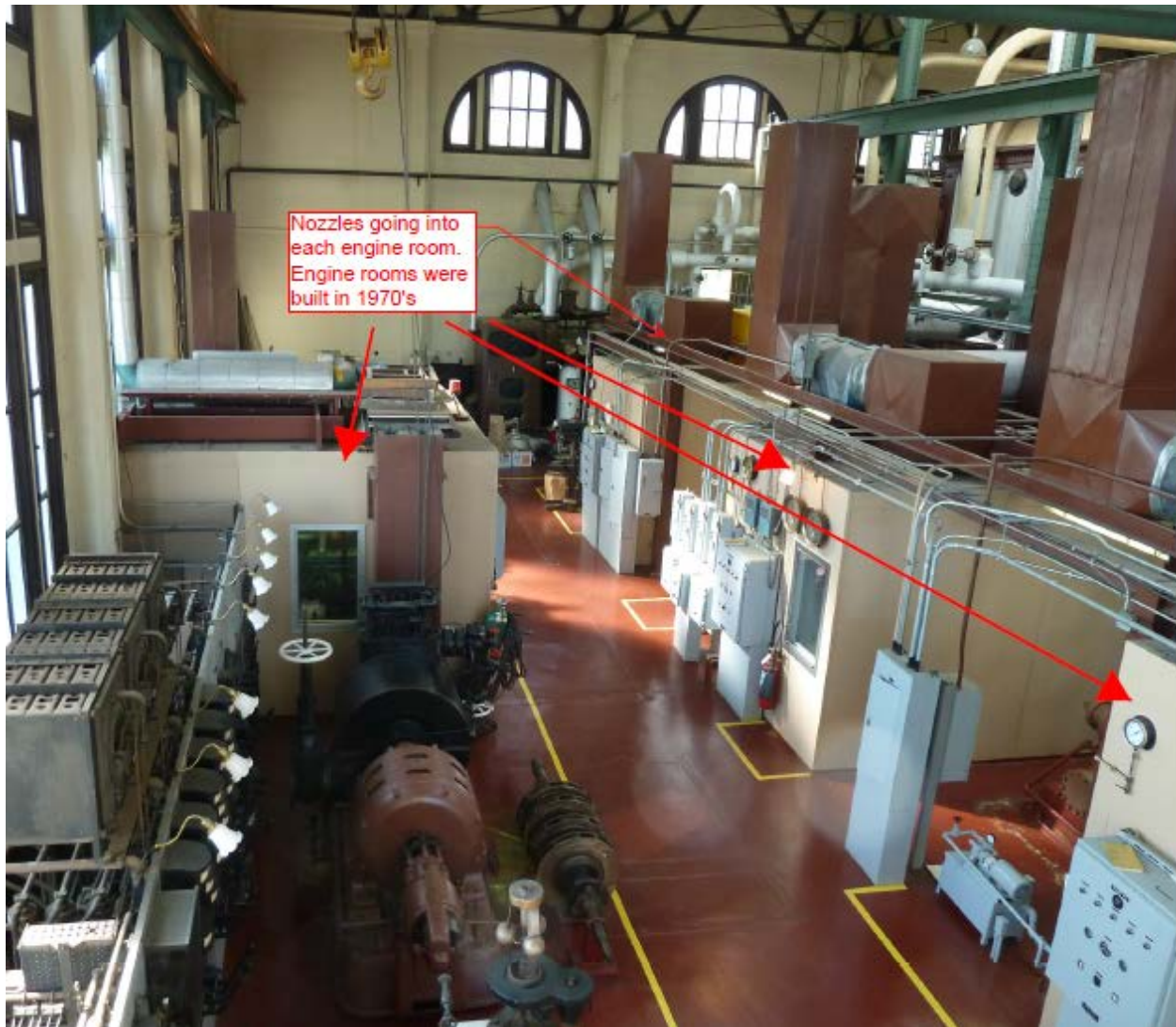
FIGURE 23 - Existing conduits and utility frame.
