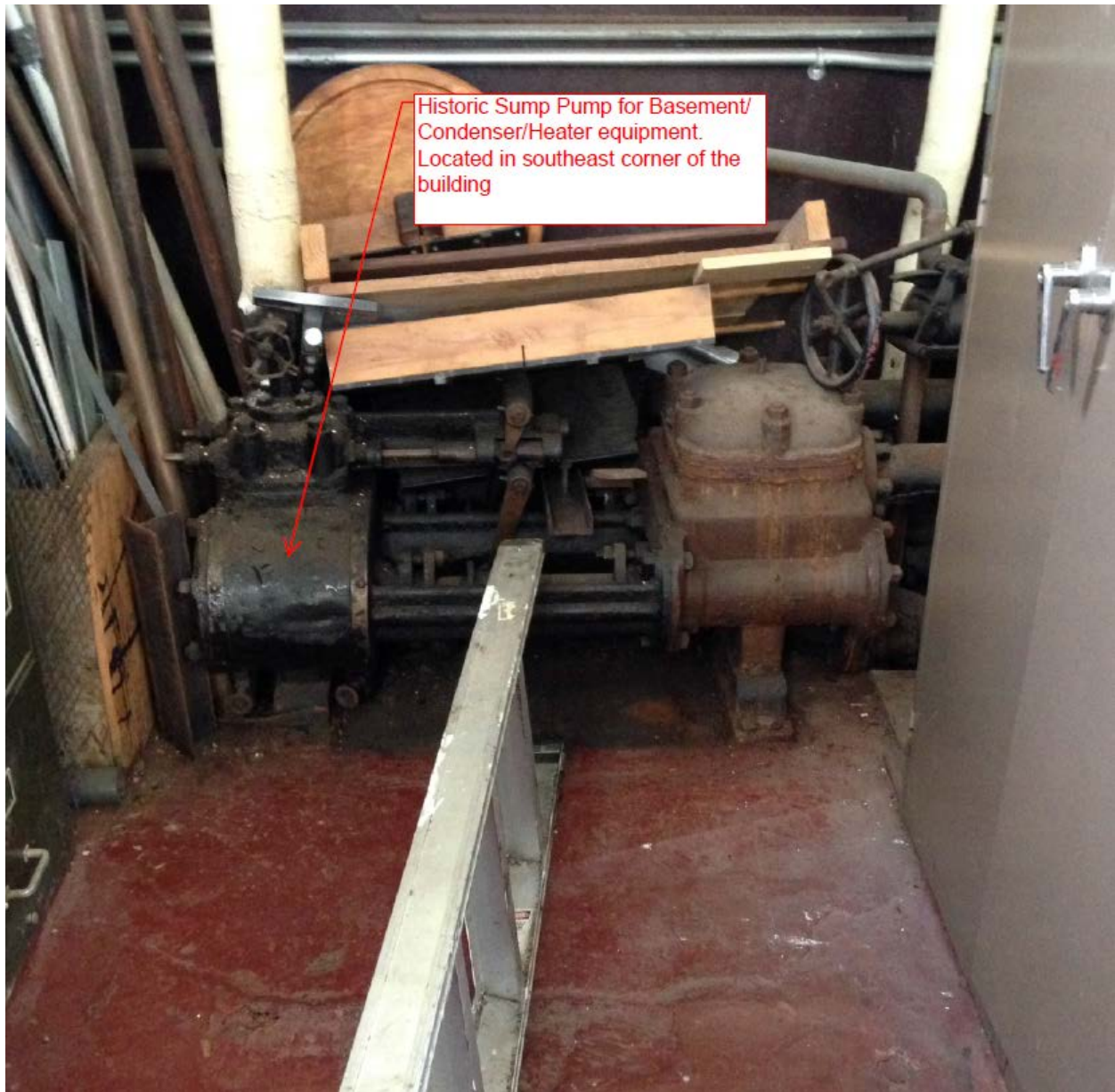
FIGURE 22 - Sump Pump in southeast corner of building.
