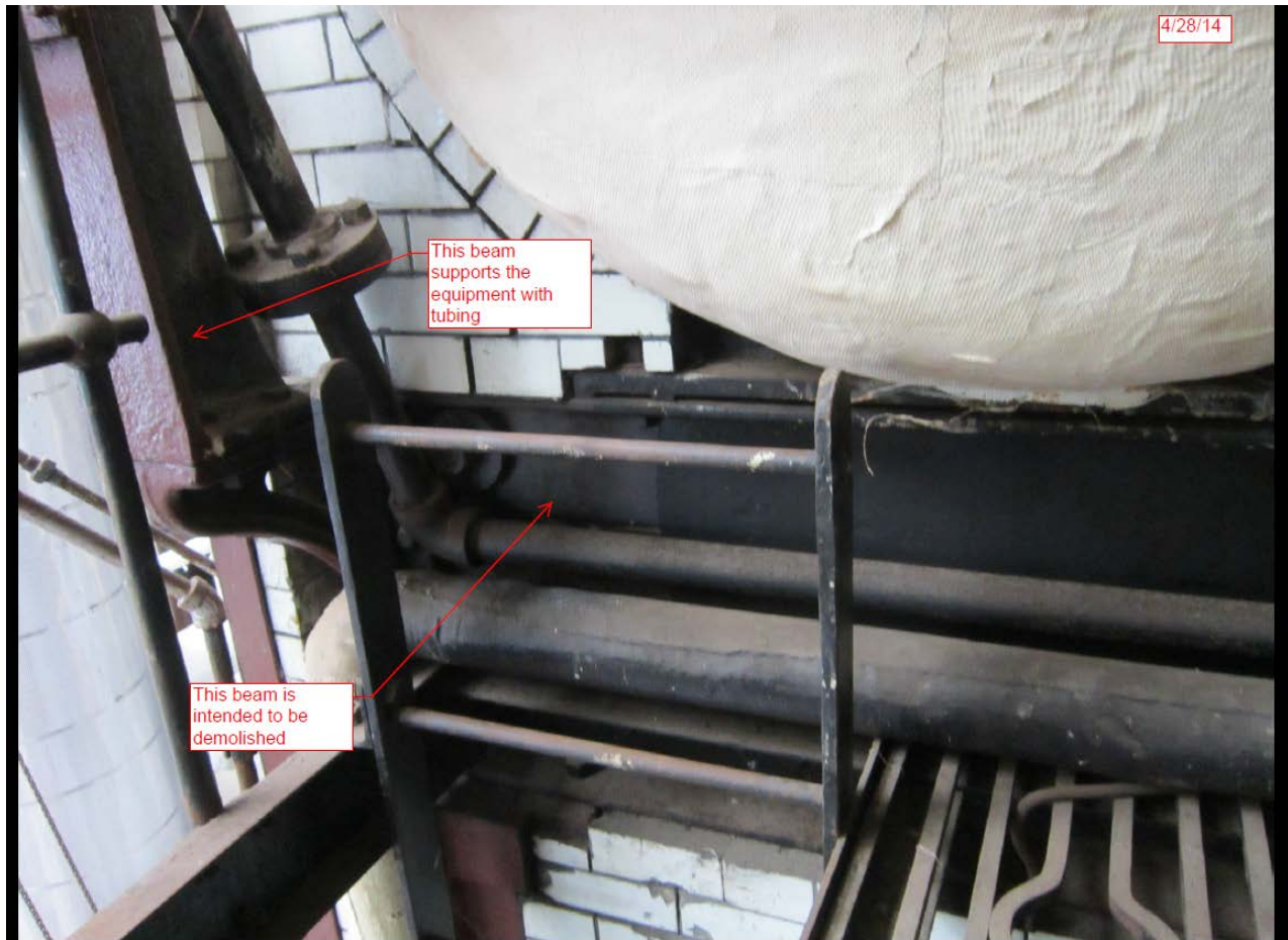
FIGURE 4 - Tubing above boiler support
