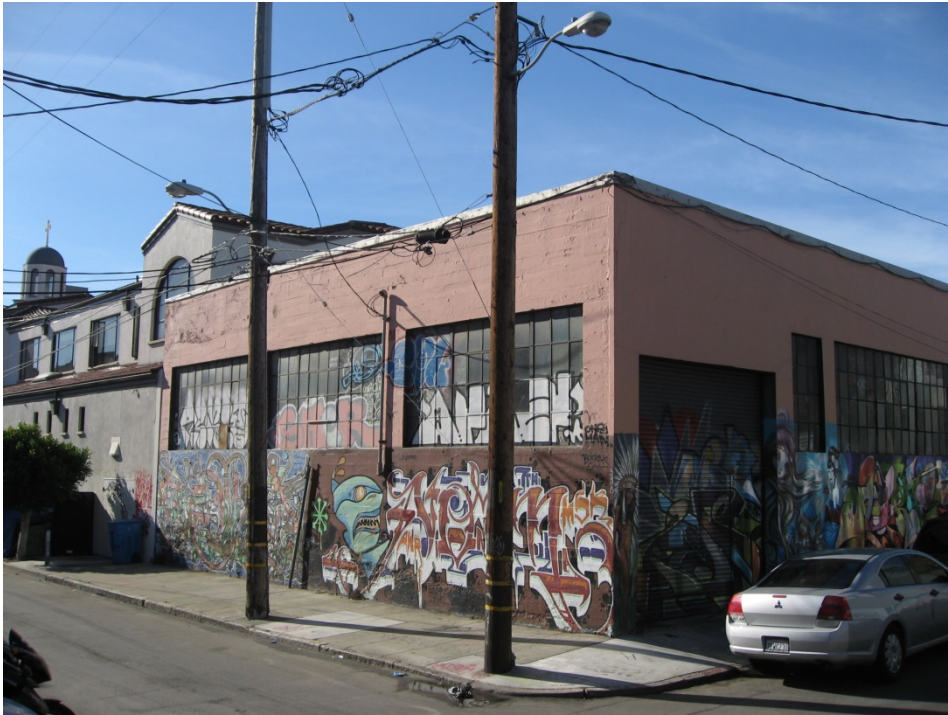
View of rear (east) facade.
