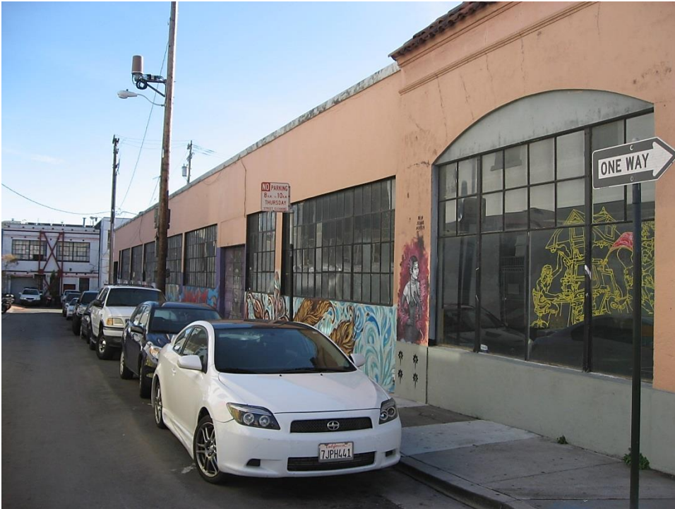
View of north facade.
