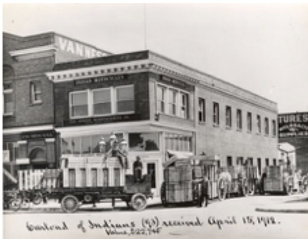
Hendee Manufacturing Company receives a delivery of Indian Motorcycles at 234 Van Ness Avenue, April 18, 1912.
