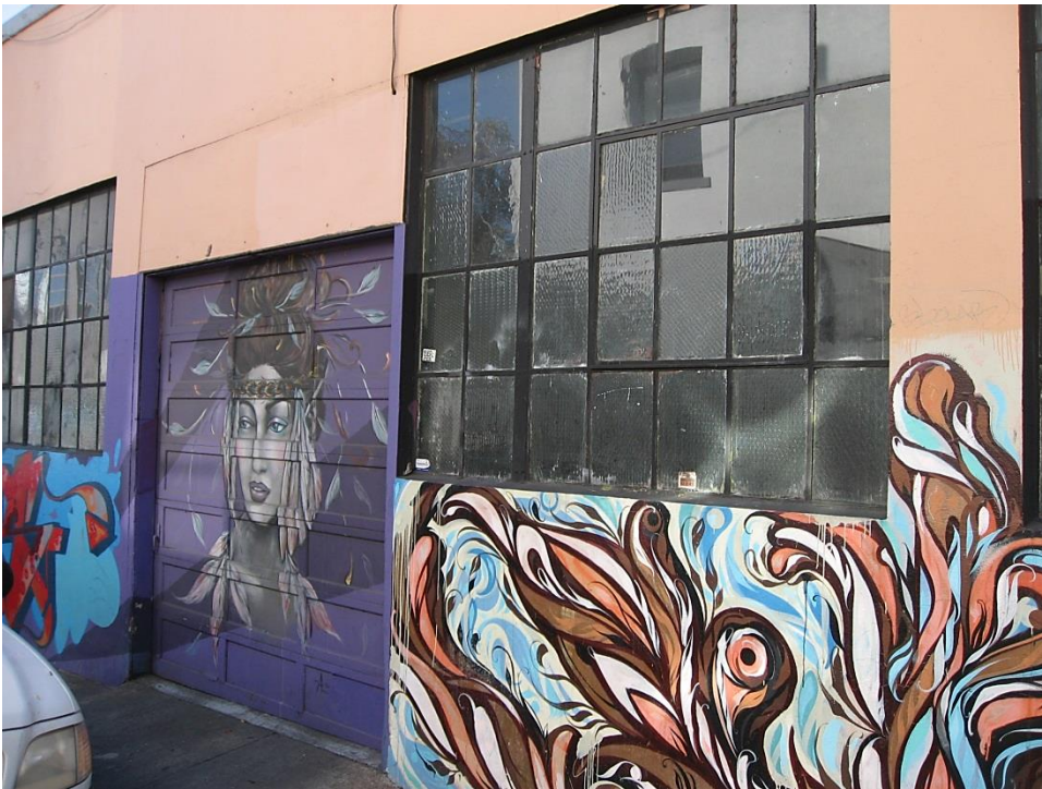
Detail of windows on north facade.
