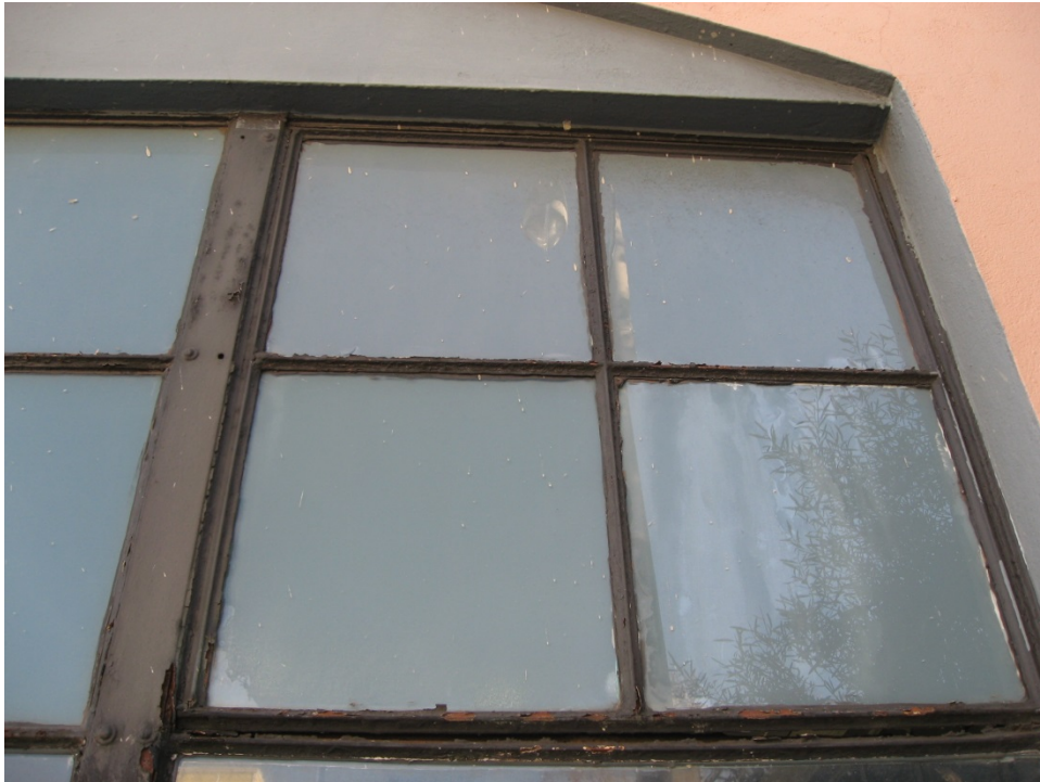
Detail of steel-sash window on primary facade.
