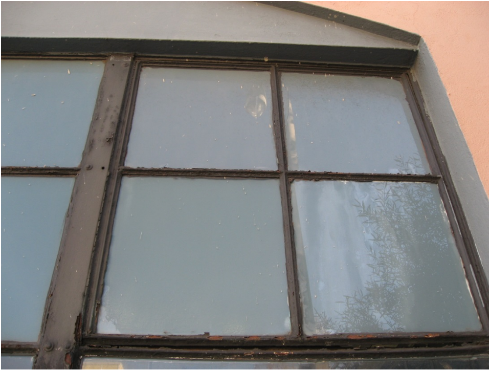
Detail of steel-sash window on primary facade.
