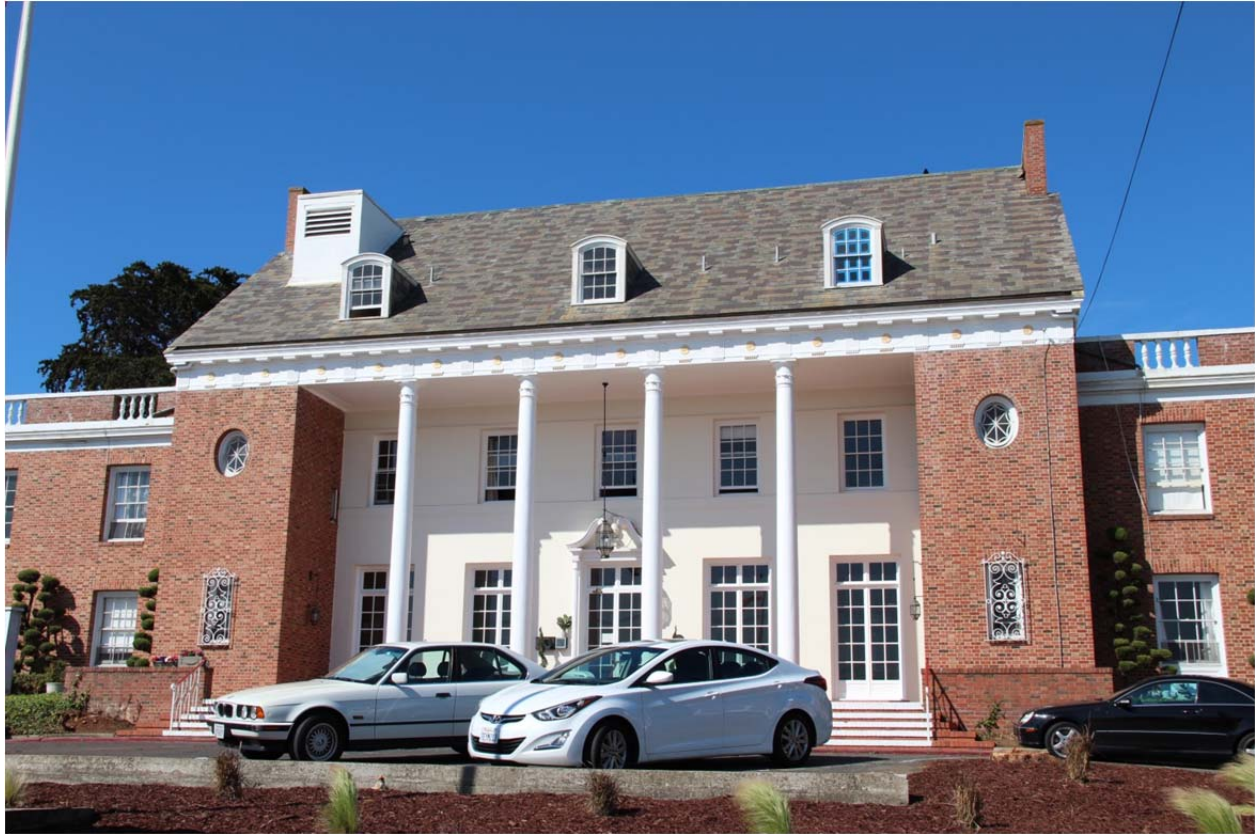
Primary façade of main building, April 2015
