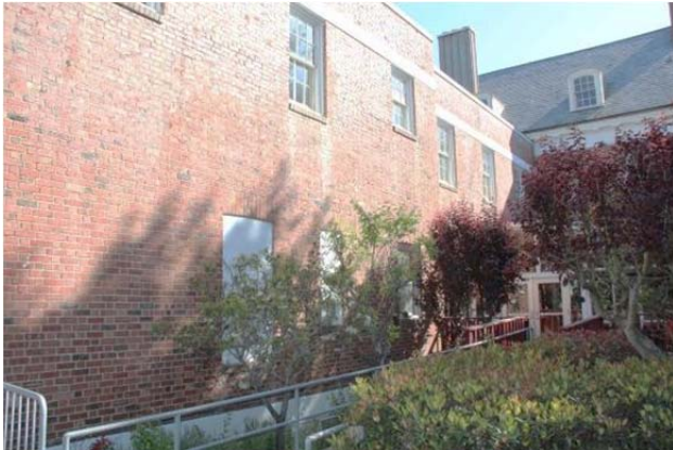
South elevation of service wing, April 2015
