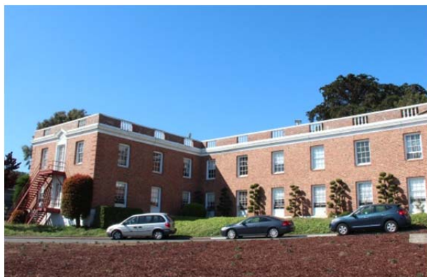
Primary (east) façade of south wing, April 2015
