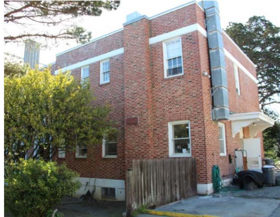
North elevation of service wing, April 2015
