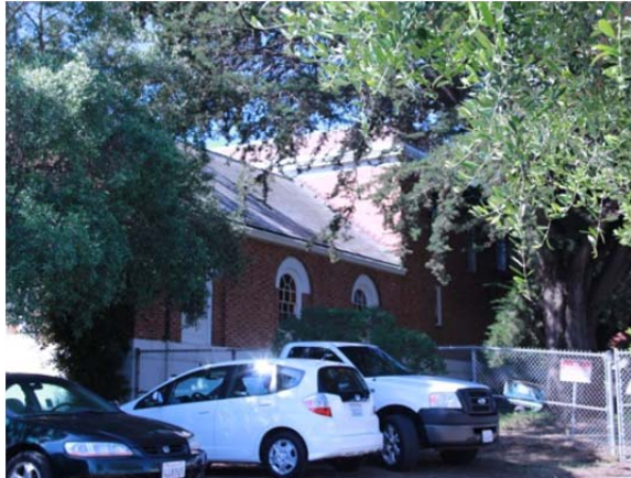
North elevation of chapel, April 2015
