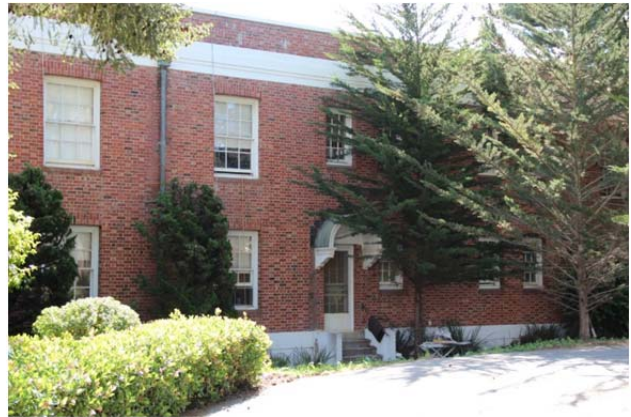
West elevation of south wing, April 2015
