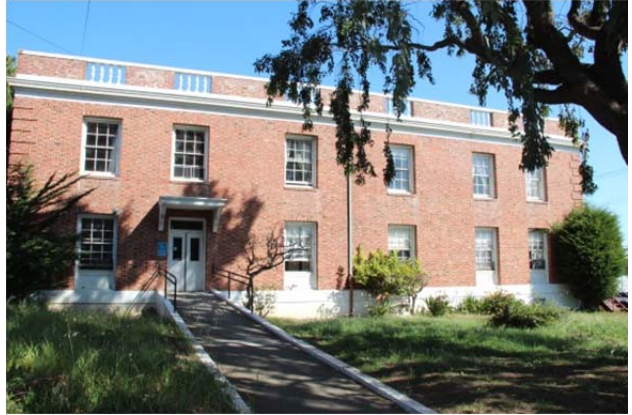
South elevation of south wing, April 2015
