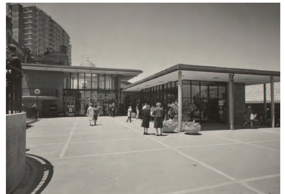
View looking west from Fountain Plaza, 1960s (Environmental Design Archives)
