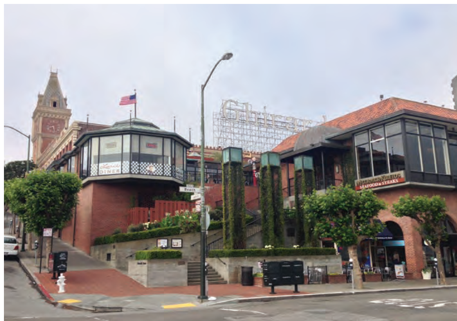
View looking southwest at Larkin and Beach streets
