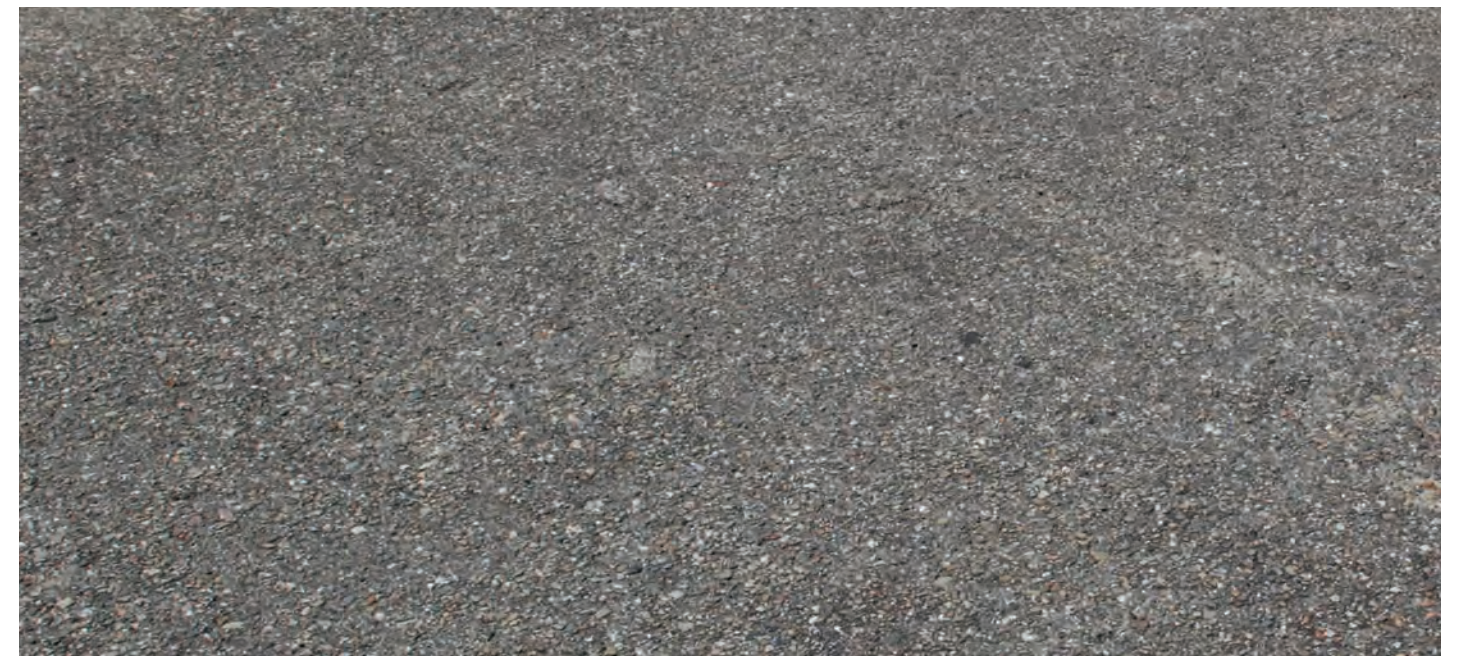
New paving to match original paving in color, texture, and material
