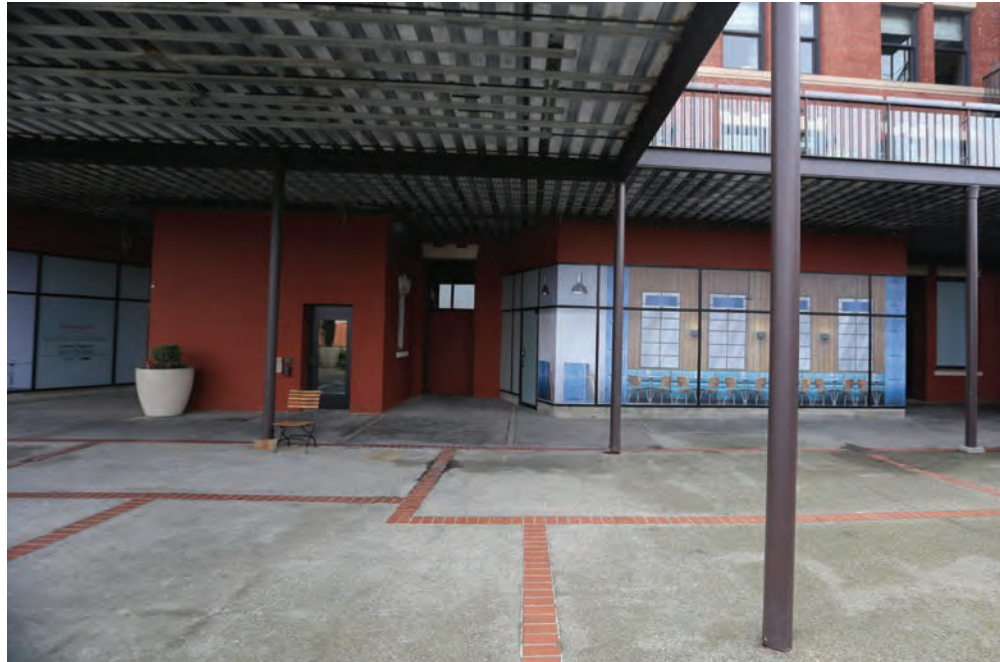
Existing image of storefront enclosure at the Mustard Building, north facade
