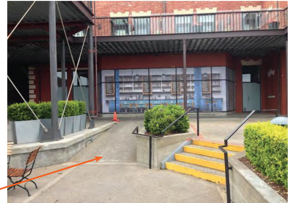
Stairs at Terrace Plaza, looking south towards Mustard Building
