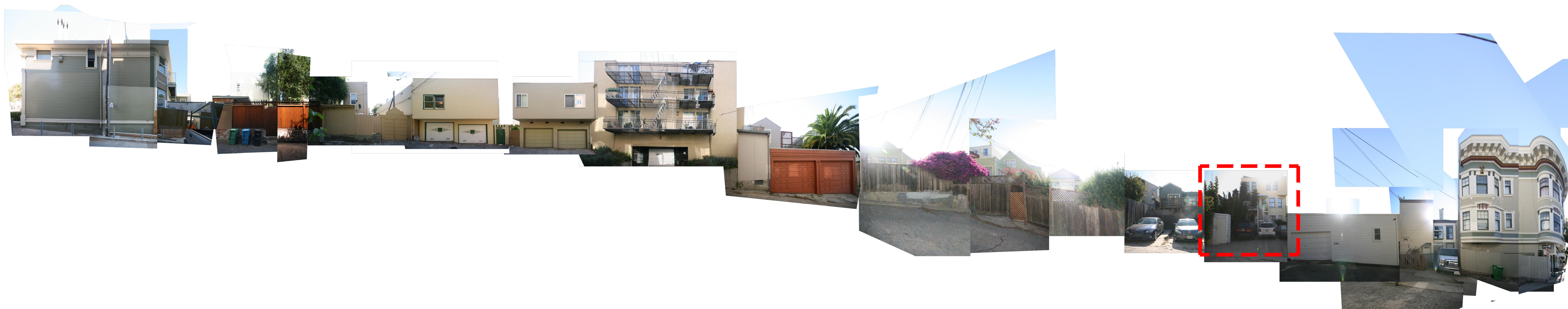
3 AMES STREET – REAR FACADE
