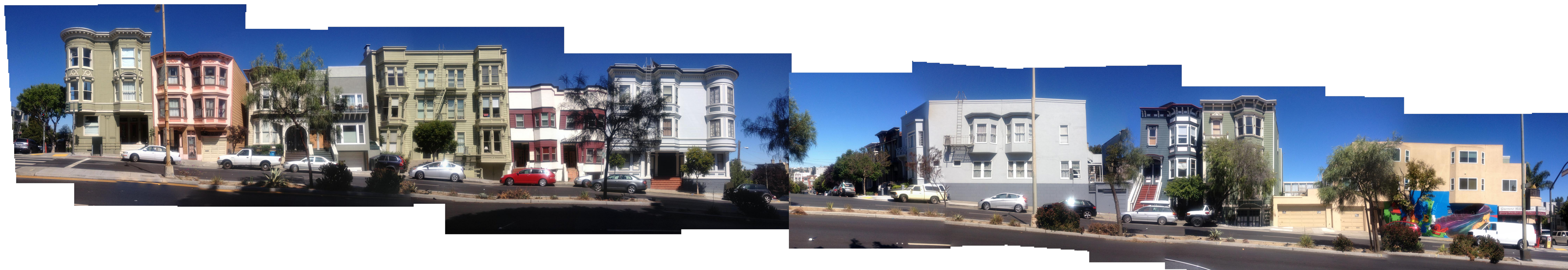
2 GUERRERO STREET LOOKING EAST – OPPOSITE FACE OF STREET
