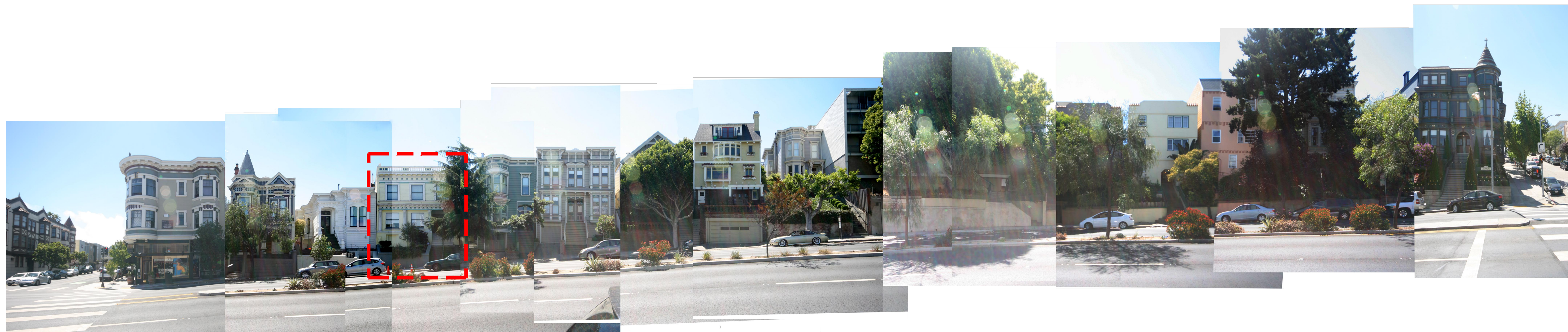
1 GUERRERO STREET LOOKING WEST – FRONT FACADE
