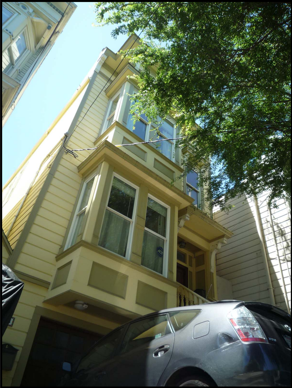
918 Minnesota Street, January 2015 (Source: Applicant)
