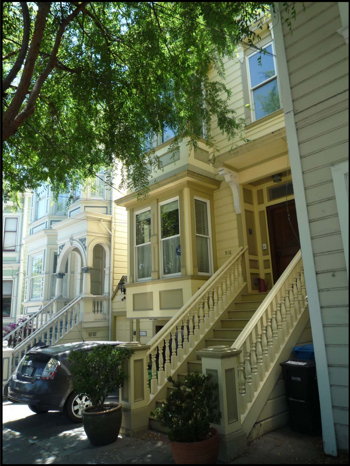
918 Minnesota Street, January 2015 (Source: Applicant)
