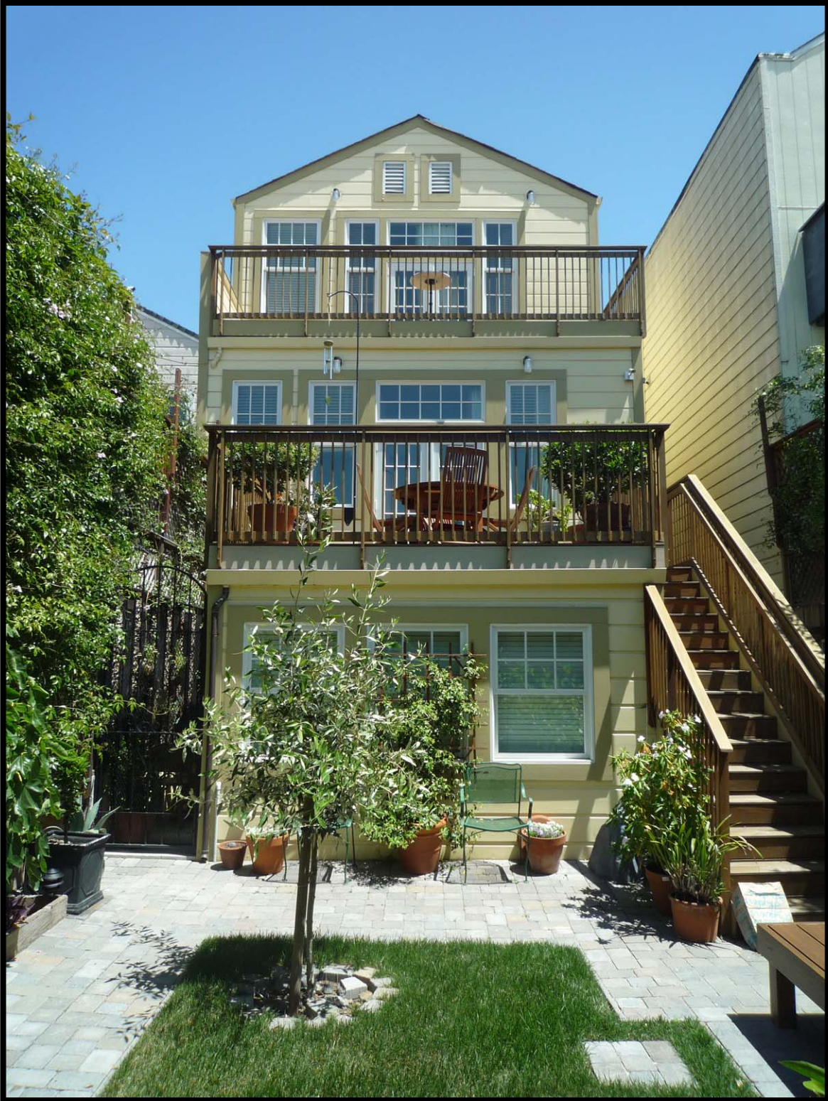
918 Minnesota Street, Rear Facade, January 2015 (Source: Applicant)
