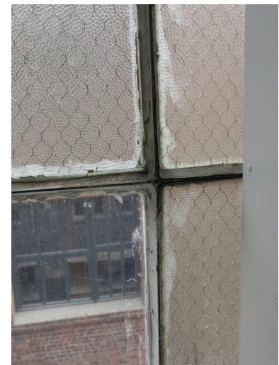
WIRED GLASS AT REAR WINDOWS
