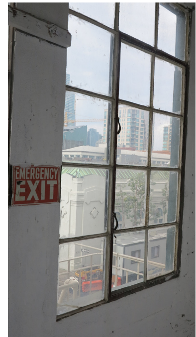
FRONT WINDOW AT FIRE ESCAPE (CASEMENT)
