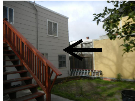
VIEW OF BLDG DIRECTLY TO THE WEST
