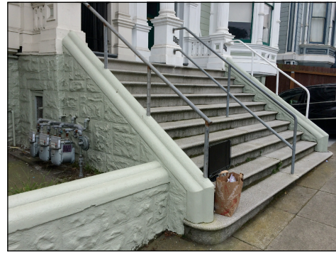
EXISTING ENTRY STAIRS
