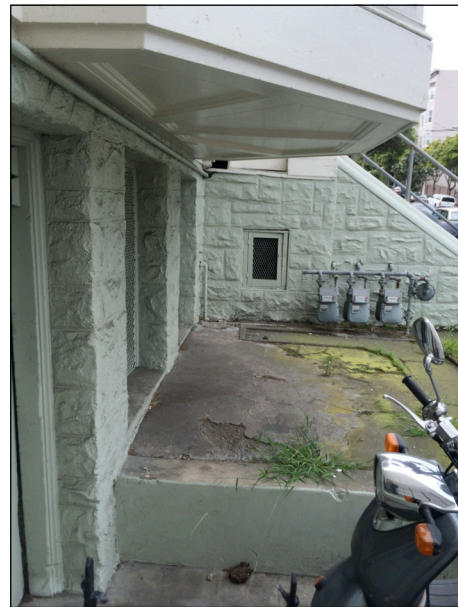
EXISTING FACADE PROFILE
