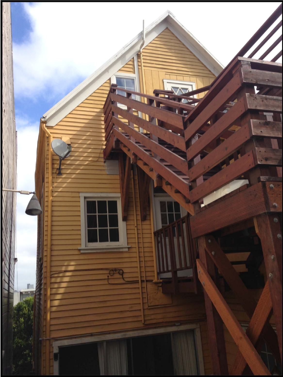
3751-3752 20 th Street, Rear Facade (Source: Planning Department)
