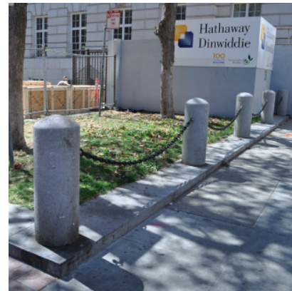
Granite bollards with chain along McAllister St east of Federal Building
