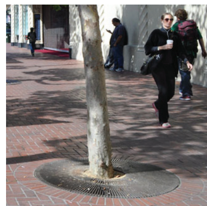
Circular tree well with radial metal tree grate along Market St
