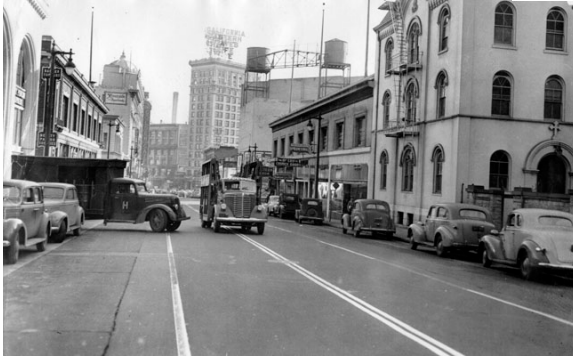
Figure 1.2-2: View along Golden Gate Avenue of Subject Building in 1944, Center-Right. Source: San Francisco Public Library Photo Collection.
