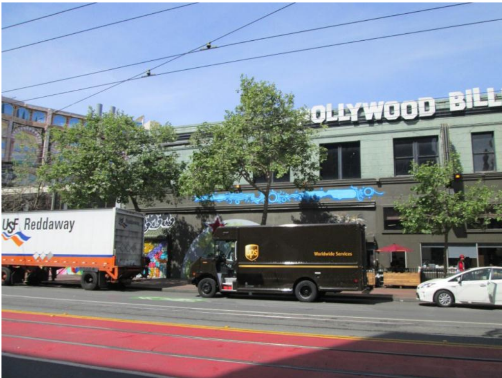
A-4: GOLDEN GATE BUILDING, SOUTH ELEVATION, WEST END
