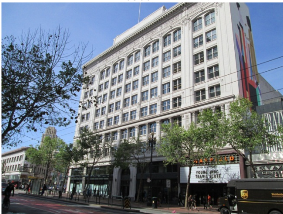
Figure 1.3-13: Loew's Warfield Theatre Building, Looking north.
