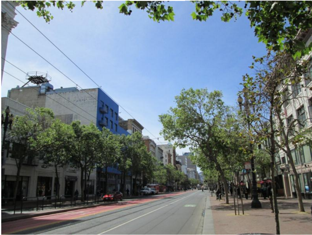
A-39: DISTRICT VIEWS, NEAR INTERSECTION OF MARKET AND TAYLOR, LOOKING SOUTHWEST
