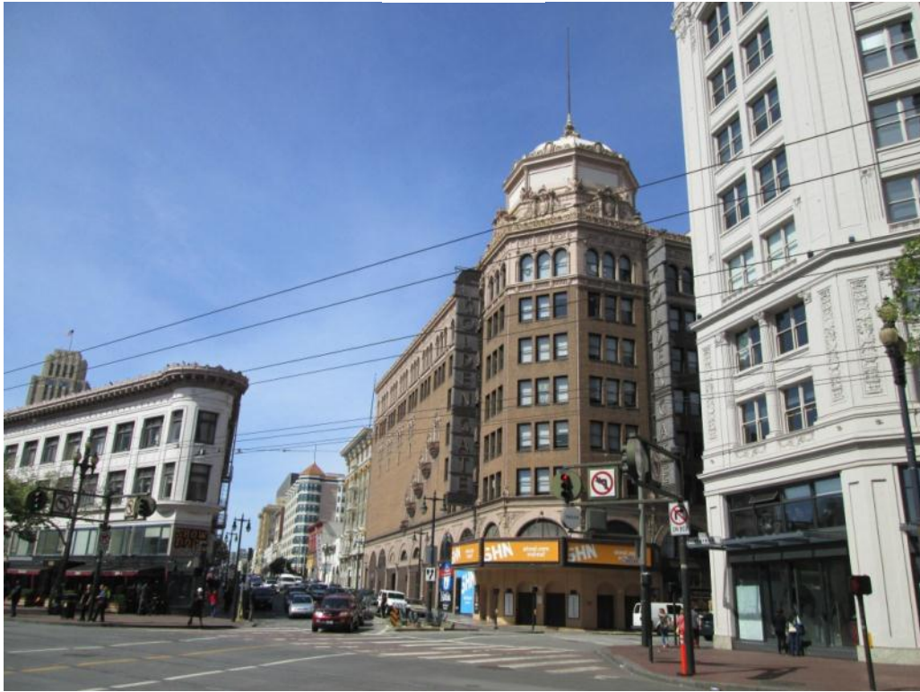
A-13: DISTRICT VIEWS, INTERSECTION OF MARKET AND TAYLOR, LOOKING NORTHWEST
