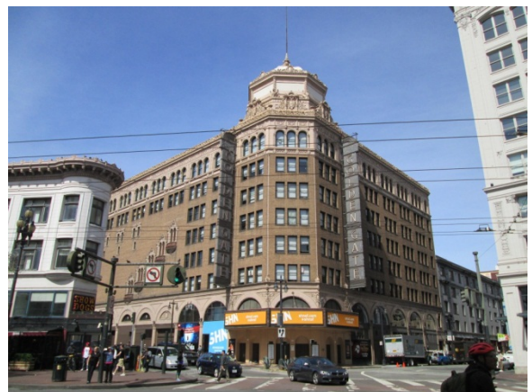
Figure 1.3-8: Golden Gate Theatre Building, Looking north.
