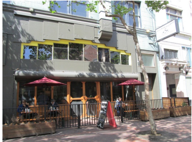
Figure 1.2-9: Looking North at East End Storefront
