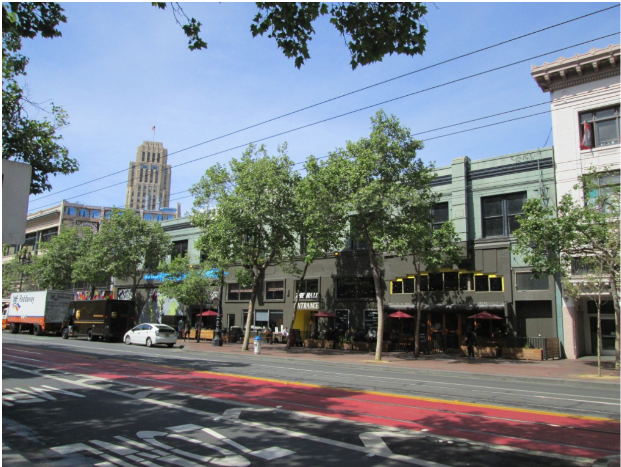
Figure 1.2-5: 1028-1056 Market Street, Looking Northwest at South Elevation
