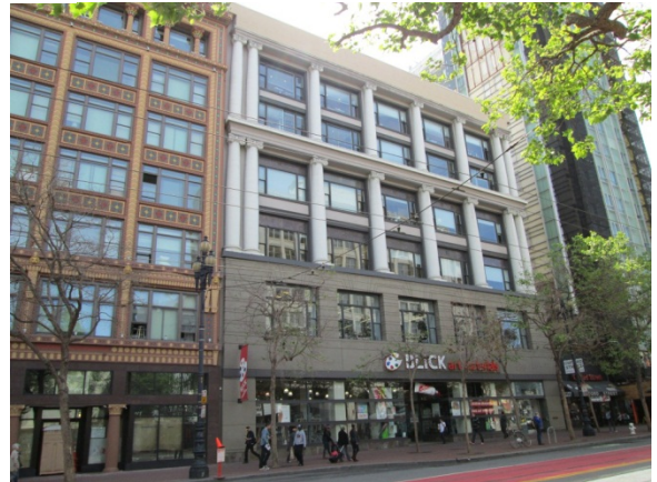
Figure 1.3-10: Hale Brothers Building, Looking south.
