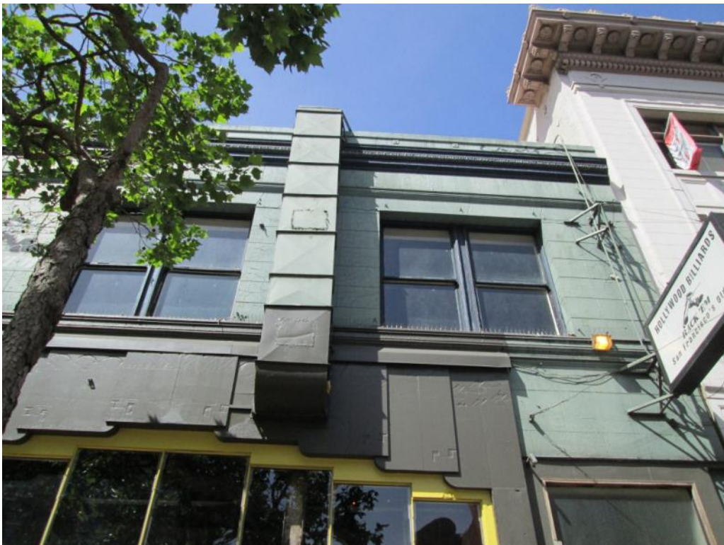
A-10: GOLDEN GATE BUILDING, SOUTH ELEVATION, EAST END, SECOND STORY
