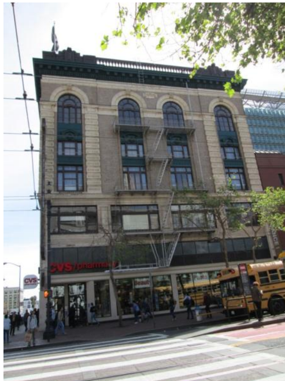
A-30: DISTRICT VIEWS, 6-26 7 TH STREET, LOOKING SOUTH
