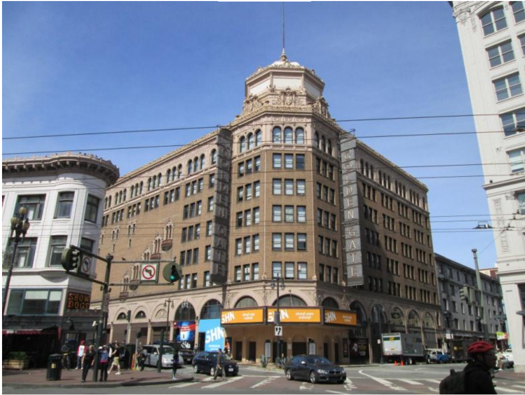
A-15: DISTRICT VIEWS, GOLDEN GATE THEATRE, 1-35 TAYLOR, LOOKING NORTH
