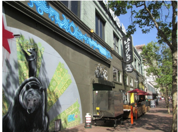
Figure 1.2-7: Looking Northeast at West End Storefront
