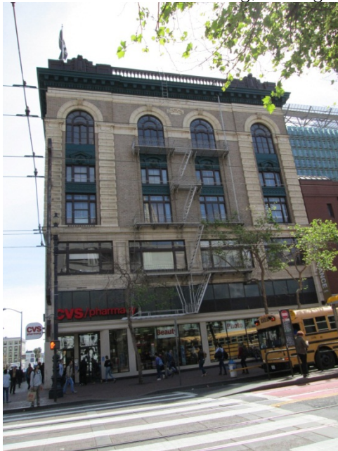
Figure 1.3-11: Odd Fellows Hall Building, Looking south.
