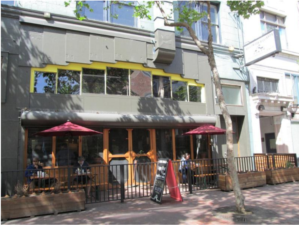
A-9: GOLDEN GATE BUILDING, SOUTH ELEVATION, EAST END, FIRST STORY
