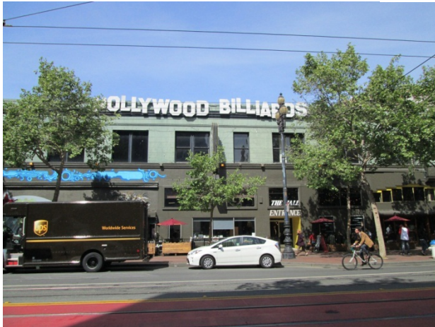
Figure 1.2-6: Looking North at Center of South Elevation
