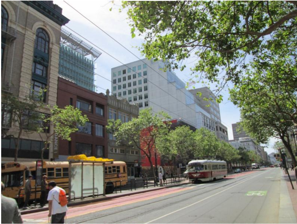
A-29: DISTRICT VIEWS, WEST END OF DISTRICT, LOOKING SOUTHWEST
