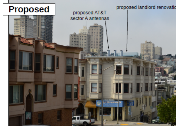
Previously approved AT&T Mobility “Macro” WTS Facility in Telegraph Hill. Three faux vent pipes (with three antennas) on roof, and equipment inside the garage.
