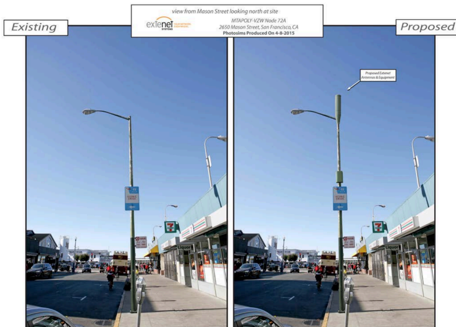
Extenet Systems, for Verizon Wireless “oDAS R” (or Small Cell) on a steel light pole owned by the SF Public Utilities Commission. An antenna is located on top and two computers (equipment) are located midway down the pole. Planning Department staff worked with the Department of Public Works, and the carrier to create a bracket to “screen” one of the computers with road signage.
