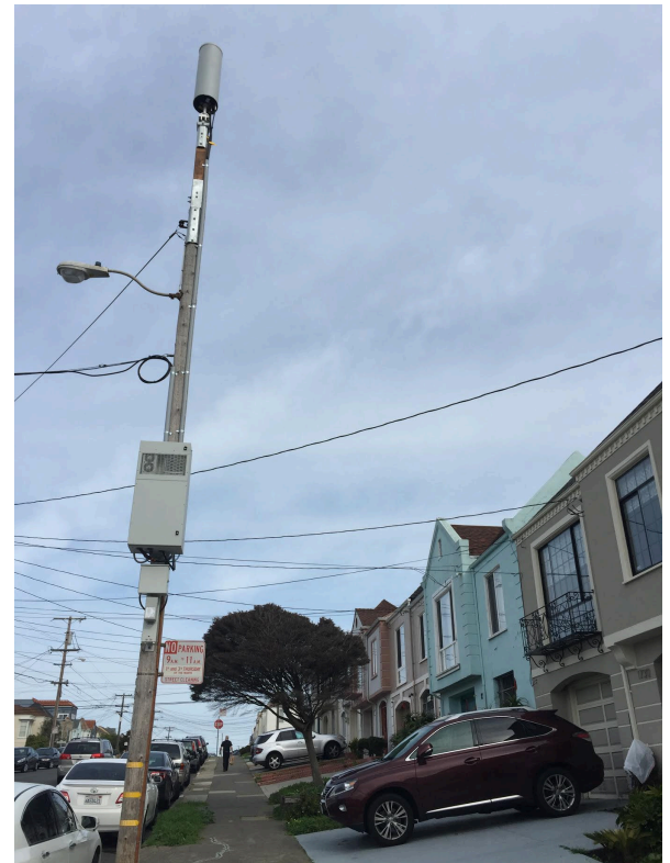
Crown Castle, for Verizon Wireless, “oDAS XL” in the Outer Sunset. The bulky nature and noise generation from cooling fans on residential streets is disfavored.
