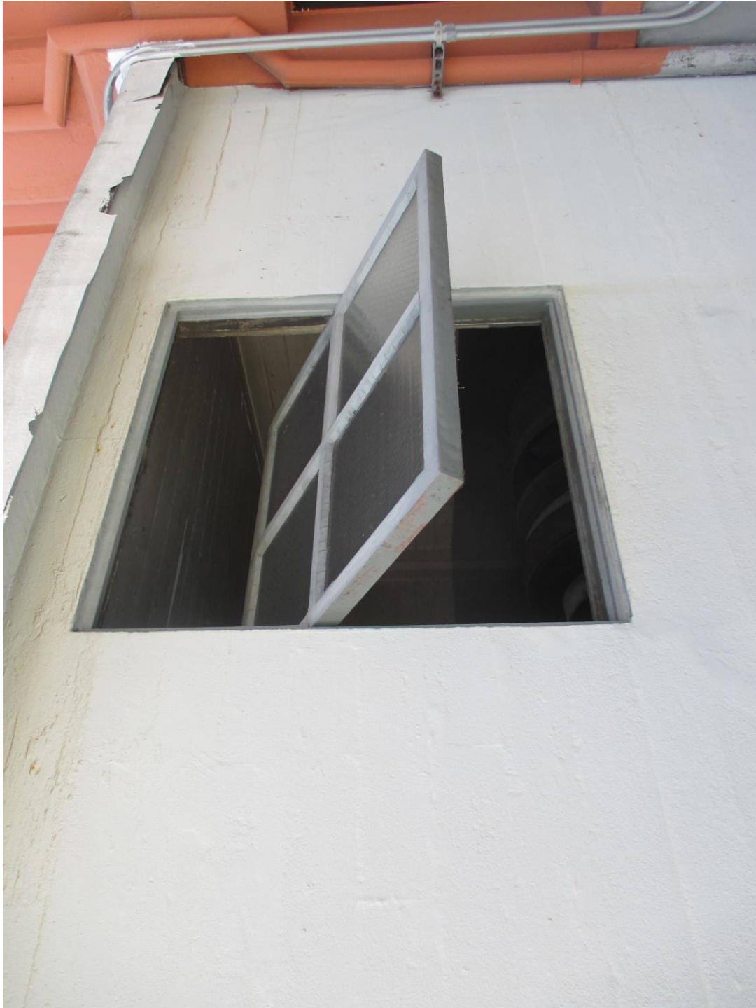
Original metal window at elevator penthouse on roof – open position
