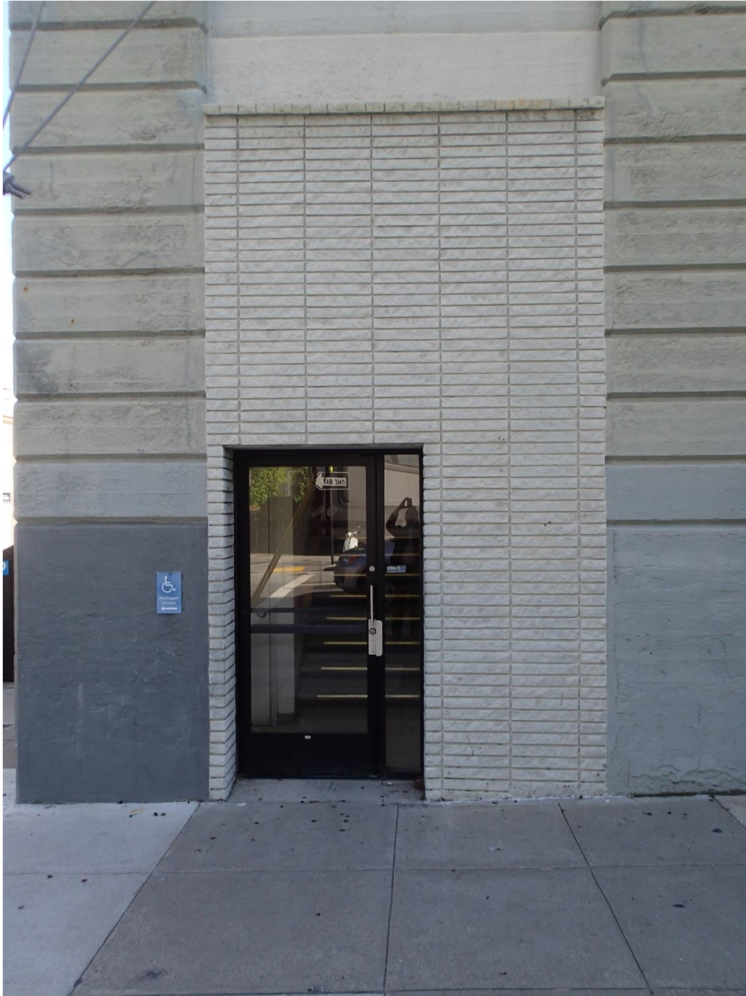
Existing Exit Door on Sansome Street (North End)
