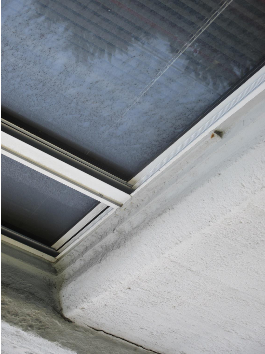
Existing replacement windows within original window frame with stops
