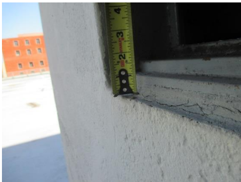
Frame width: 1" typ. + 1/2" at sill
