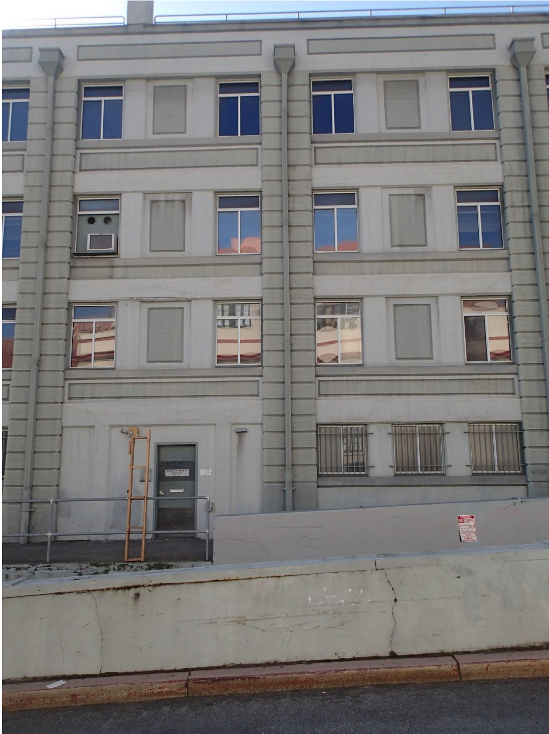
Existing North Façade on Green Street (Center Bays)
