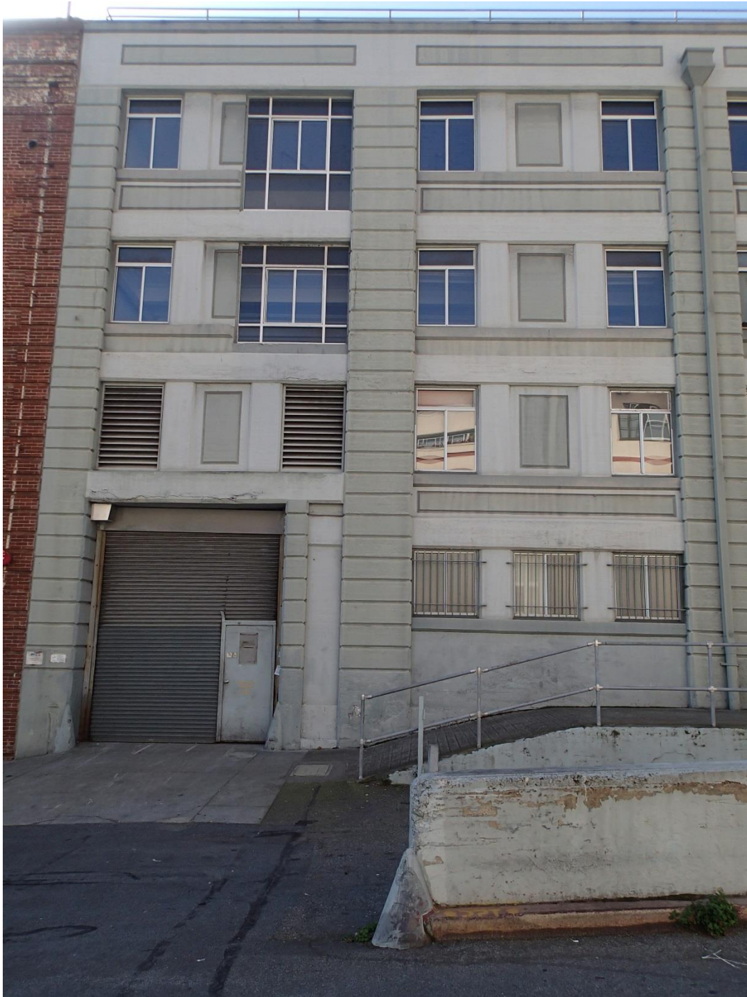
Existing North Façade on Green Street (East End)
