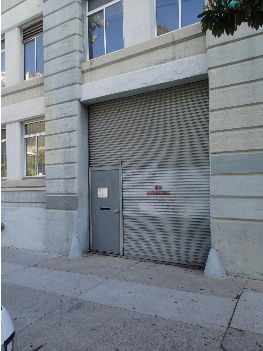
Existing Roll-Up Door on Sansome Street
