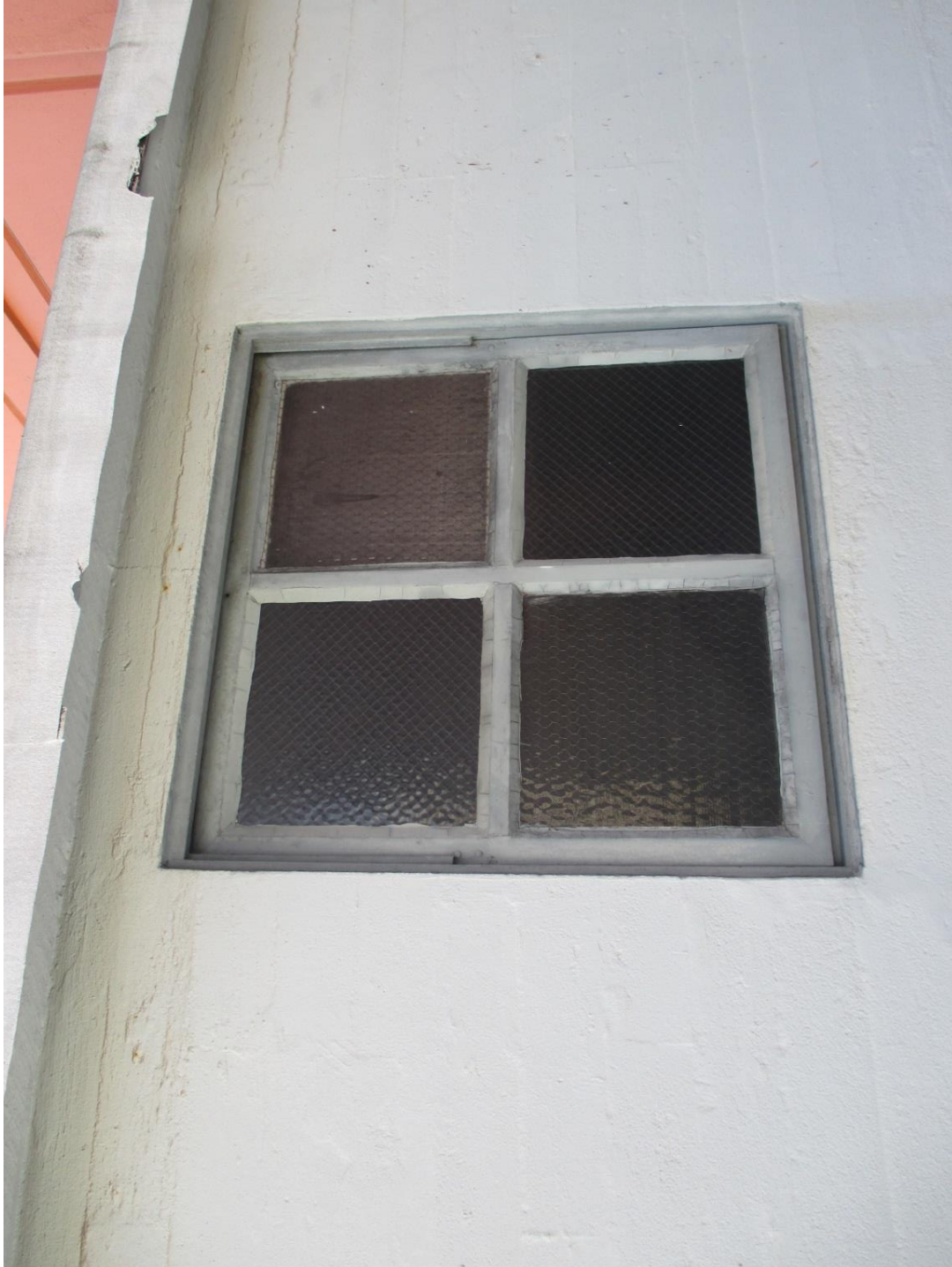
Original metal window at elevator penthouse on roof – closed position
