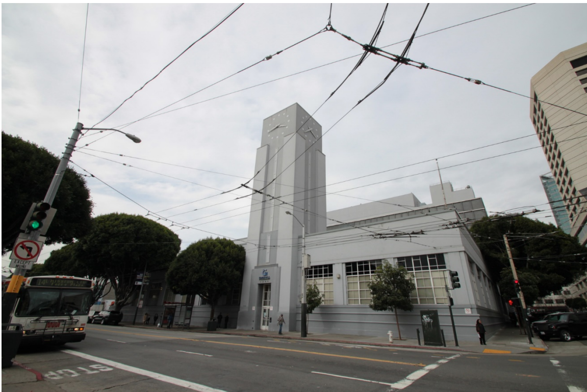
South façade, view looking northwest along Mission Street (Architectural Resources Group, January 2015)
