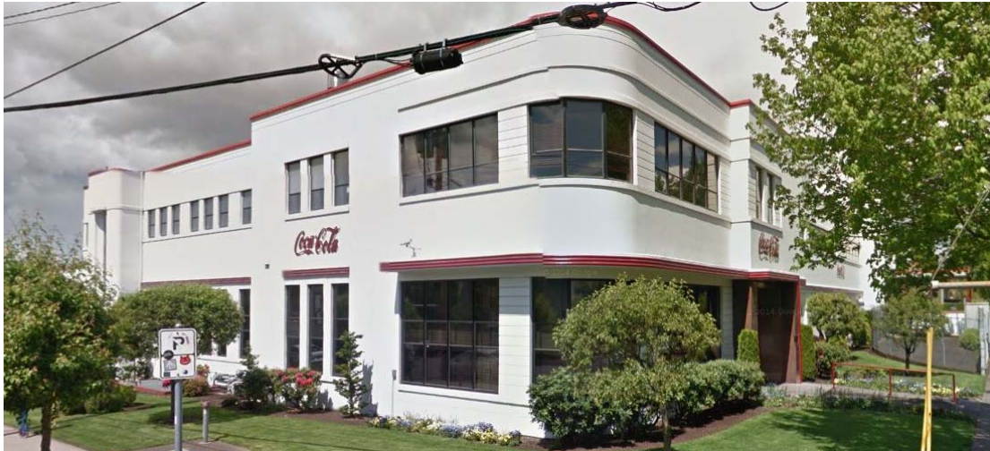
Figure 19. Portland Bottling Plant, c.1941 (southeast corner, Google Street View, 2015).
