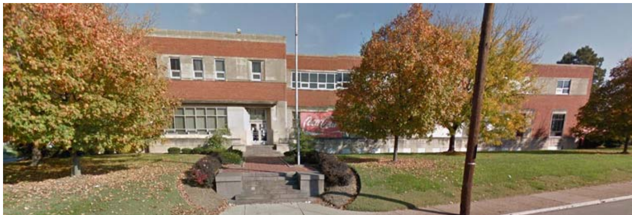
Figure 22. Louisville Bottling Plant, 1941 (front elevation, Google Street View, 2015).
