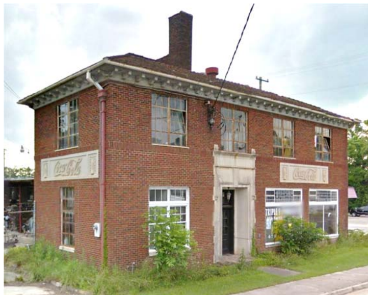
Figure 9. Coca-Cola bottling plant, Swainsboro, GA; based on standardized plan model #3 (Photo: Google Maps Street View)
