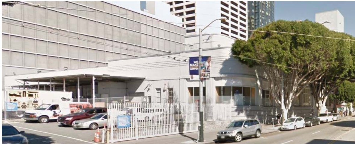
Figure 14. 1500 Mission Street, current view (Google Street View, February 2015).
