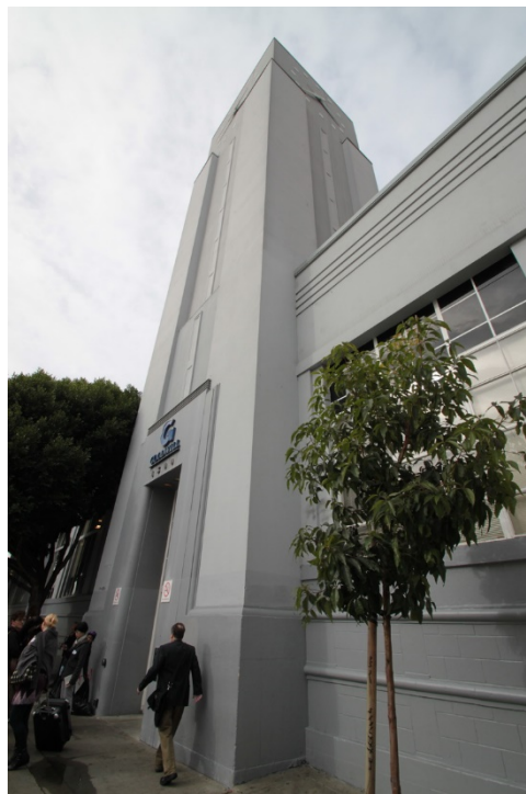
South façade, view looking west on Mission Street (Architectural Resources Group, January 2015)
