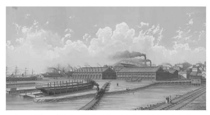
**Figure 5.** 1880s view of Union Iron Works showing the early development of the waterfront and Building 113 before it was connected in 1914. This view fails to show the plate shop at the head of the slipways. Note the bridge access to the yard along 20th Street. Bancroft Library, University of California at Berkeley.
