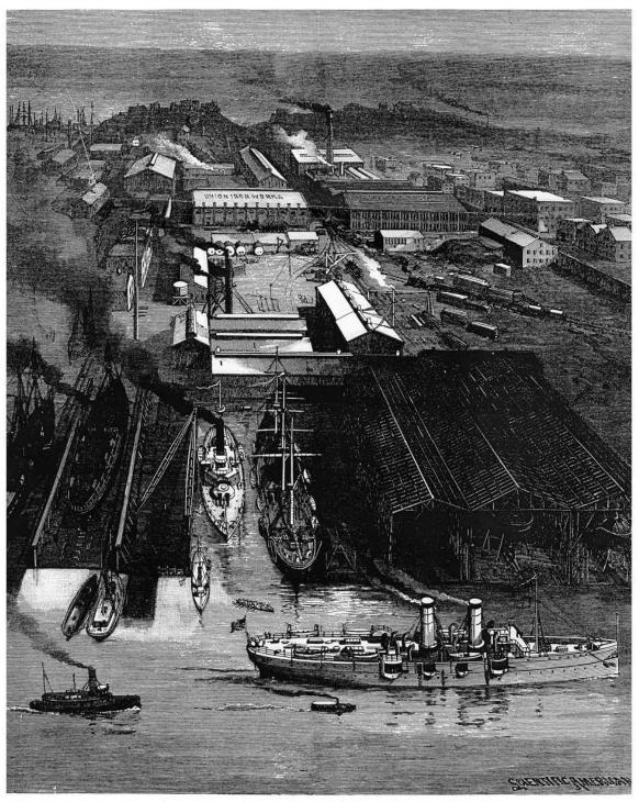
**Figure 7.** 1892 Scientific American View of the Union Iron Works Shipyard. This view shows the plate shop, the hydraulic dry dock, the truss structures and cranes over the slips, and the storage areas south of the plate shop along with the machine and metal working shops shown on earlier views.
