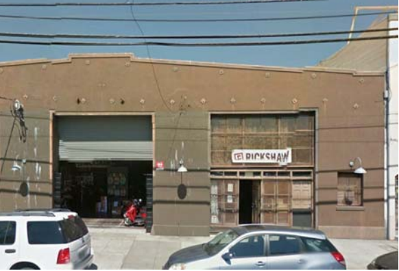
904 22nd Street with metal cornice detail and large roll-up ground floor entries
