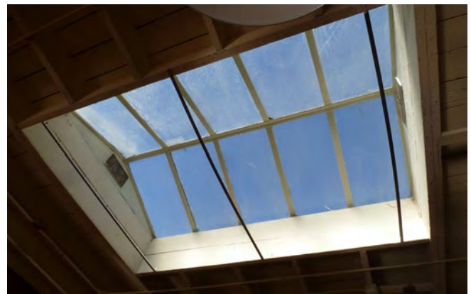
Figure 6. Skylight from interior.
