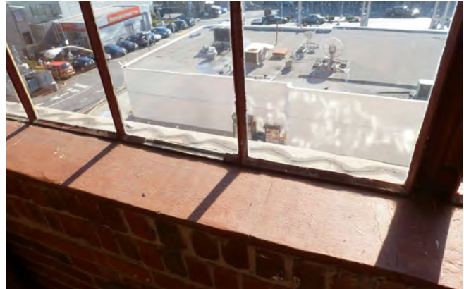
Figure 1: Window sills with concrete parge, typical.
