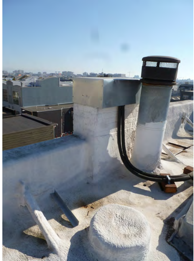
Figure 4. Capped ventilation stack and mechanical exhaust flue; note re-use of ventilation stack for services.
