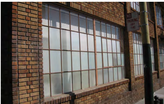
Figure 4. Typical multi-light steel windows at grade.
