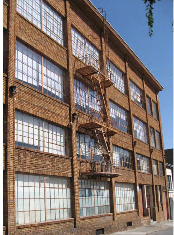
Figure 1. Metal fire escape at south elevation.
