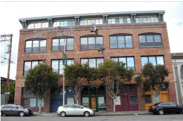
81 Langton Street (1908), converted into condominiums. (Page & Turnbull, October 2013)
