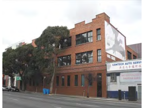
291 10 th Street, E.W. Bennett and Co. Building (1909). (Page & Turnbull, October 2013)
