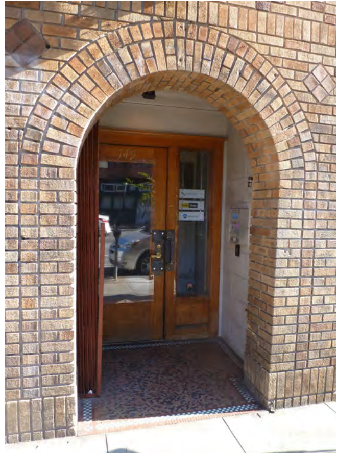
Figure 1. Entrance at northwest corner.
