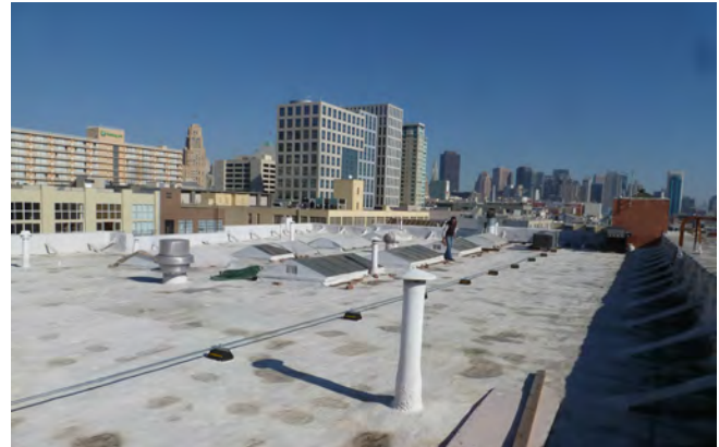
Figure 1. Roof of 149 9th Street, typical.
