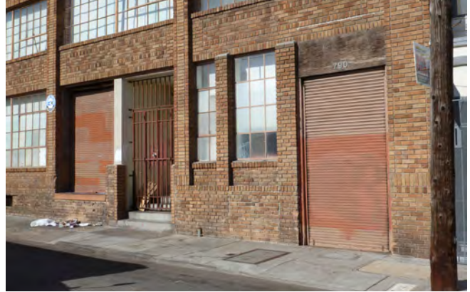
Figure 1. Service doors along south elevation.
