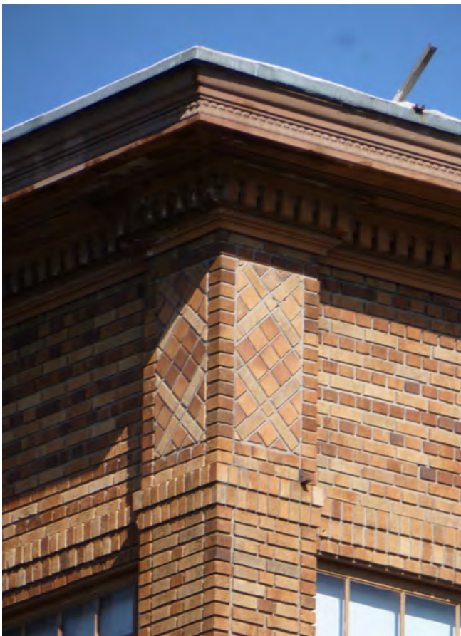
Figure 3. Southwest Corner; note decorative pattering and general brick pattern of elevation.
