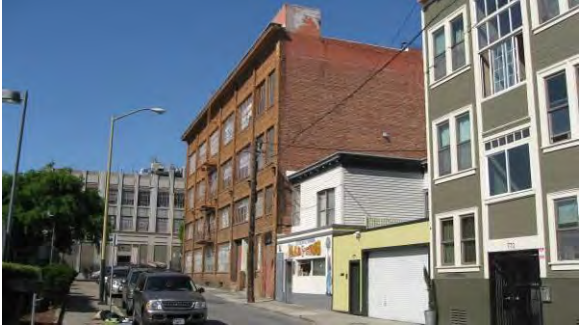
View west on Natoma Street showing a partial view of the east façade. (Page & Turnbull, April 2013)
