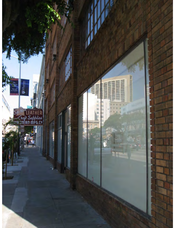
Figure 1. Typical Storefront at west elevation.
