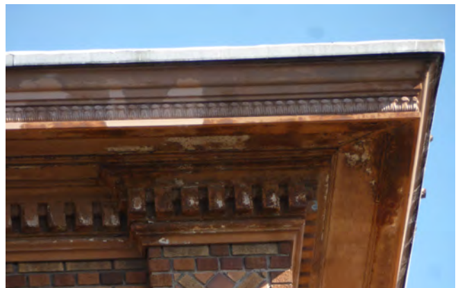
Figure 5. Cornice at southwest corner.
