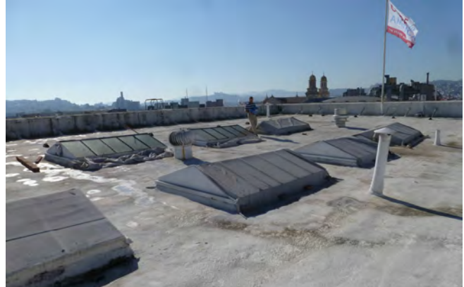
Figure 1. Roof overview; note skylights.
