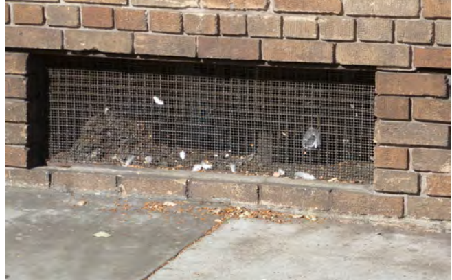
Figure 1. Ventilation grilles; note 1"x1" historic iron grille.
