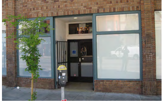
Figure 1. Storefront at west elevation.
