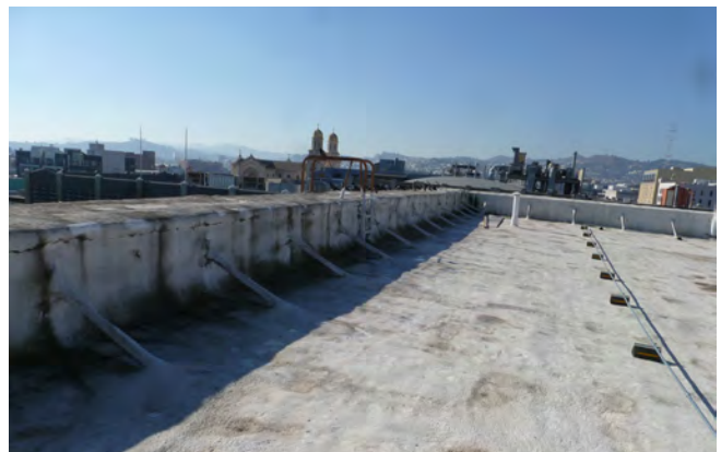
Figure 3. Parapet with bracing, typical.
