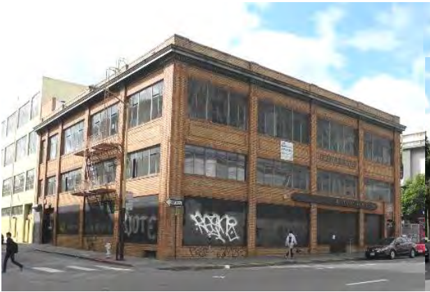
120 8 th Street, The Buzzzell Building (1925). (Page & Turnbull, October 2013)
