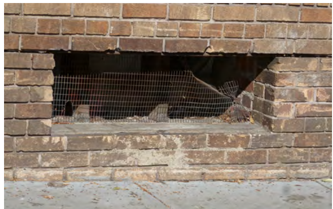
Figure 2. Ventilation grilles; replicate historic pattern from adjacent grille.
