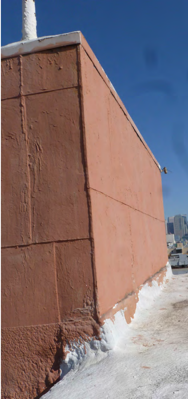
Figure 3. Enlarged view of penthouse.
