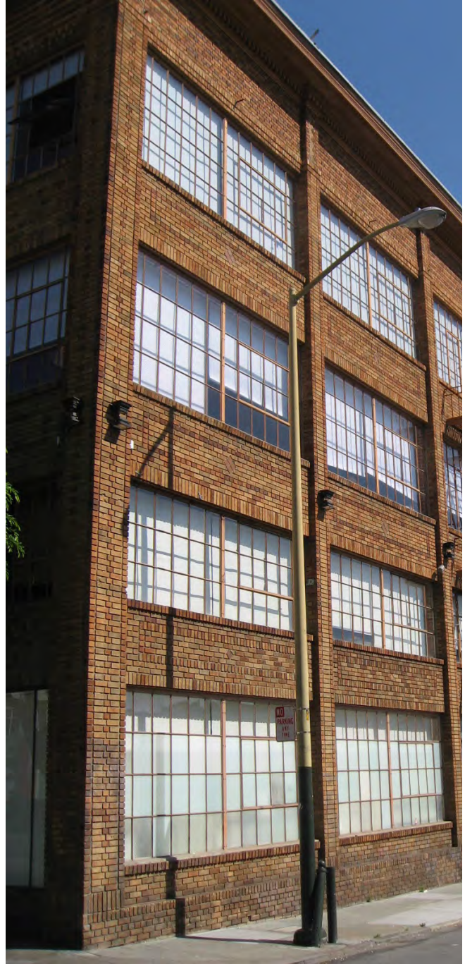
Figure 5. Typical window bay (south elevation)
