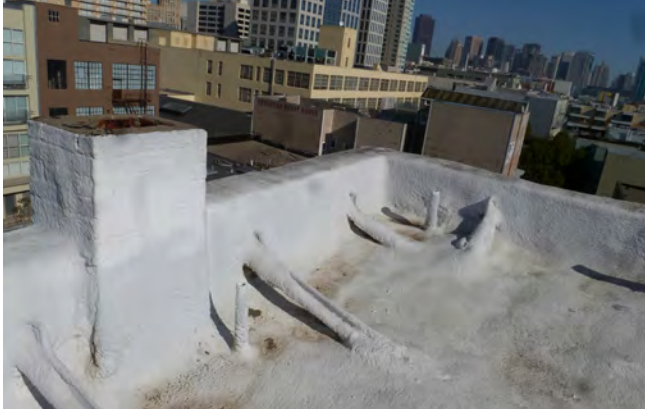
Figure 3. Roof at northeast corner, typical.
