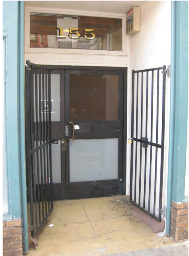
Figure 1. Metal entry door at west elevation.
