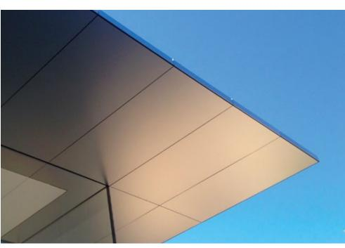
**Bead Blasted Stainless Steel Roof Overhang**Similar to South Facade Condition
