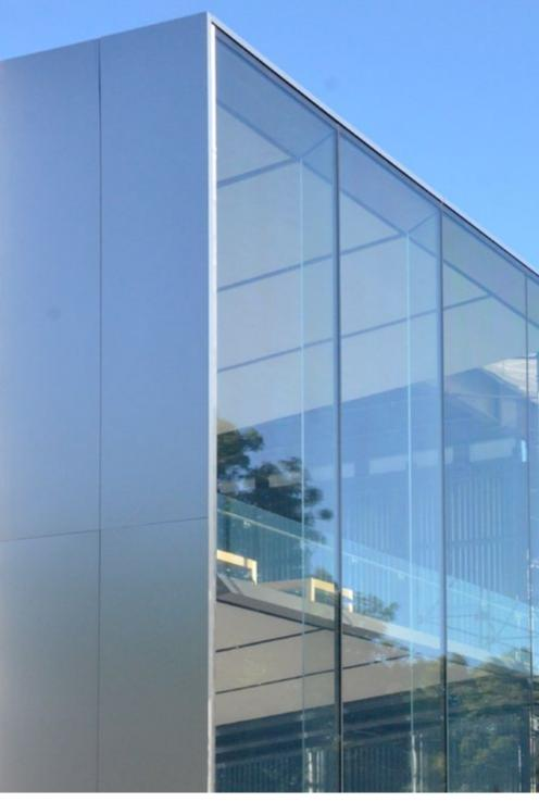
**Similar to North Facade**Bead blasted stainless steel side panels and structural glass bays
