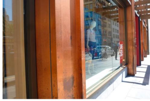
**D. Detail of the copper I-beams on the primary facade of the Levi's store.** Source: Page & Turnbull
