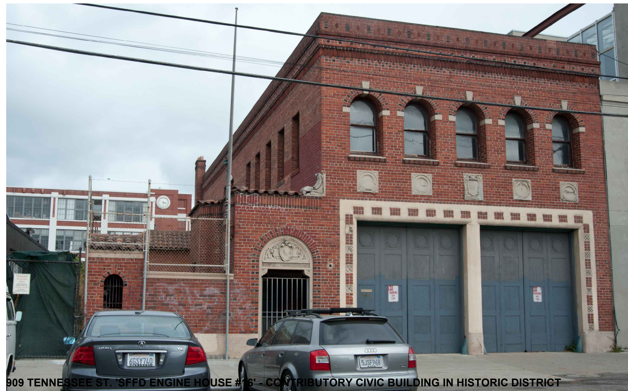
909 TENNESSEE ST. 'SFFD ENGINE HOUSE #16' - CONTRIBUTORY CIVIC BUILDING IN HISTORIC DISTRICT
