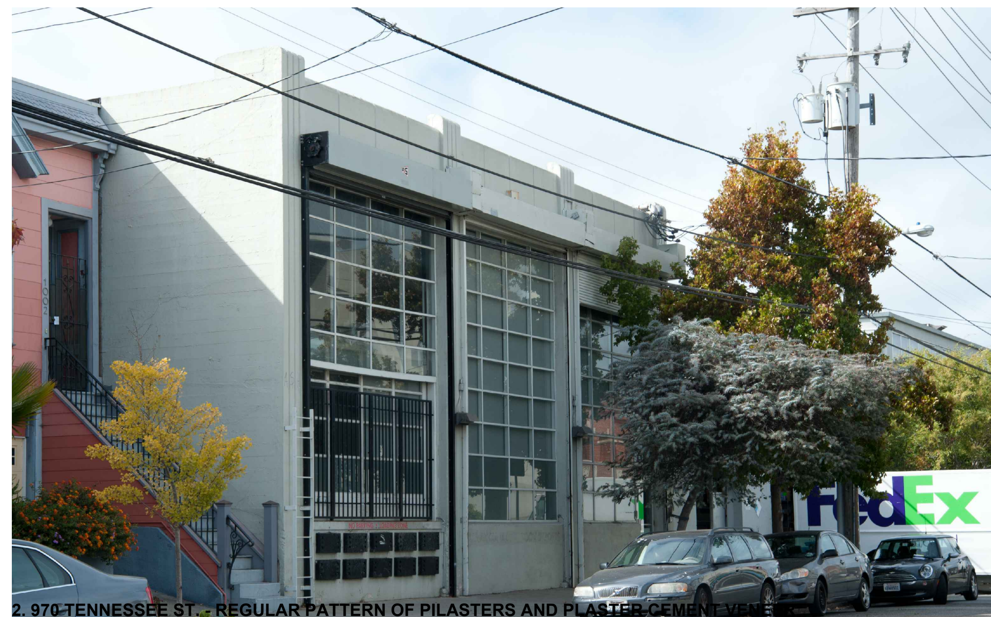
2. 970 TENNESSEE ST. - REGULAR PATTERN OF PILASTERS AND PLASTER-CEMENT VENEER
