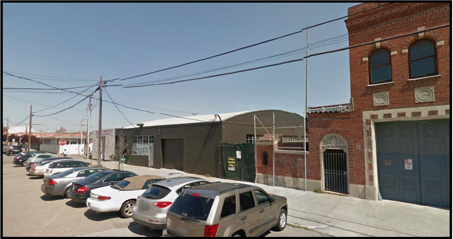
901 Tennessee Street, View along Tennessee Street, March 2014 (Source: Google Maps)
