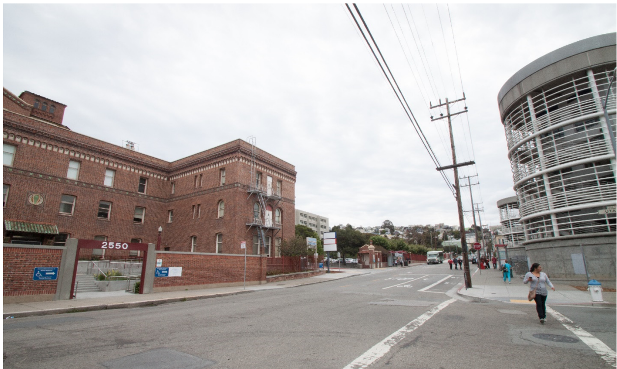
Figure 3. View of Building 9 and B/C Lot, looking east (Architectural Resources Group, August 4, 2015).
