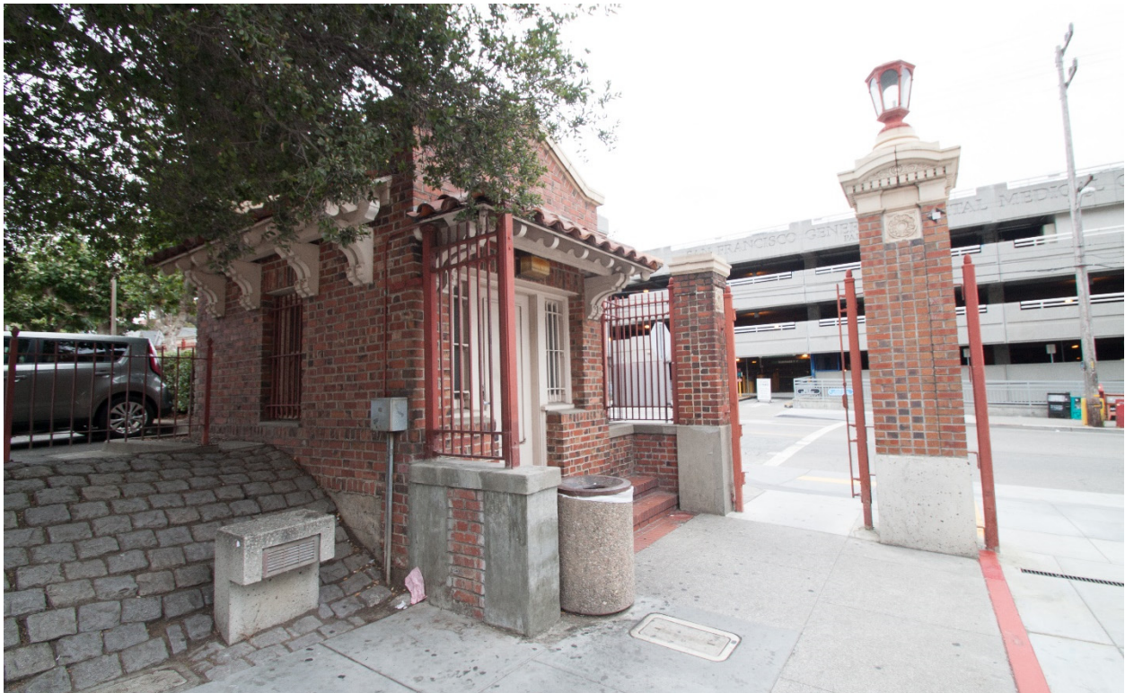
Figure 6. View of Guardhouse and Gate Pillar near southwest corner of B/C lot, looking southeast (Architectural Resources Group, August 4, 2015).
