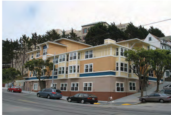
Guideline 3a: This campus residence at Parnassus Heights relates to the residential architectural vocabulary of the surrounding neighborhood.
