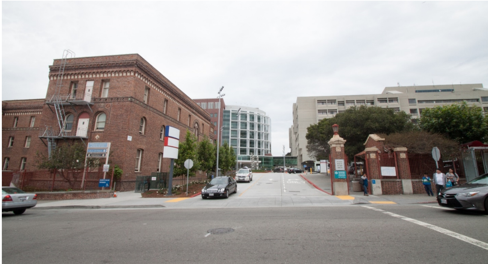
North/south access road between Building 9 and building site, looking north
