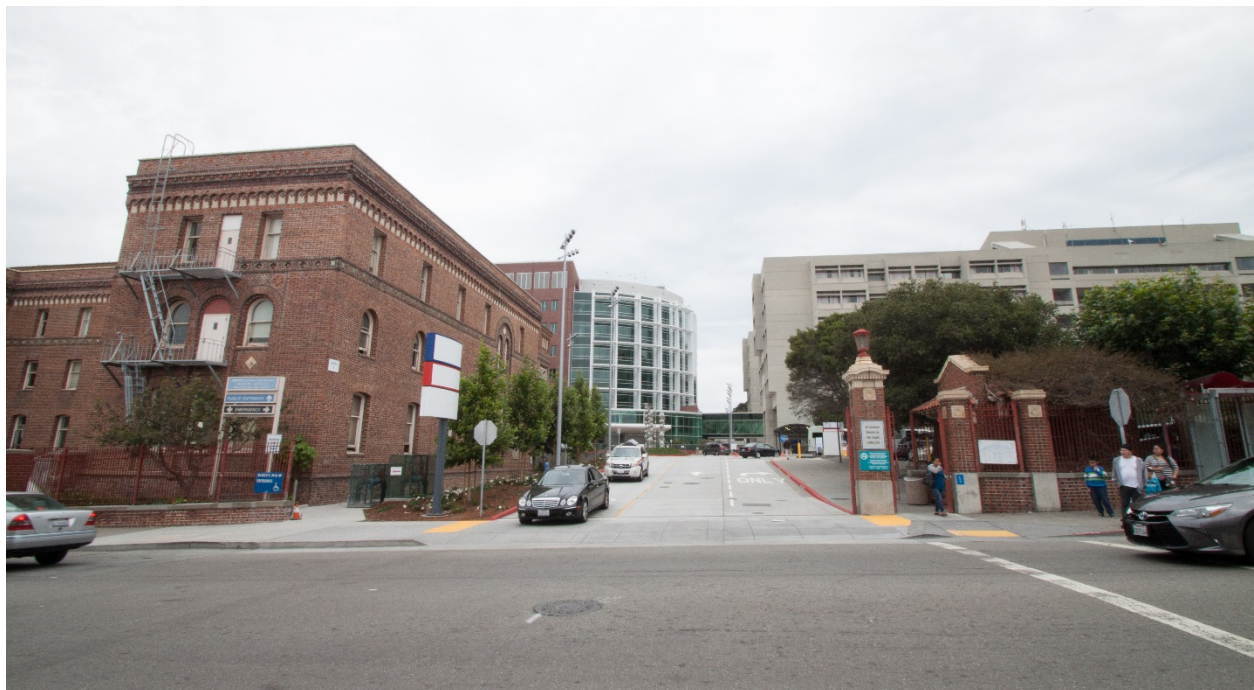
Figure 4. View of south entrance to SFGH campus, looking north (Architectural Resources Group, August 4, 2015).
