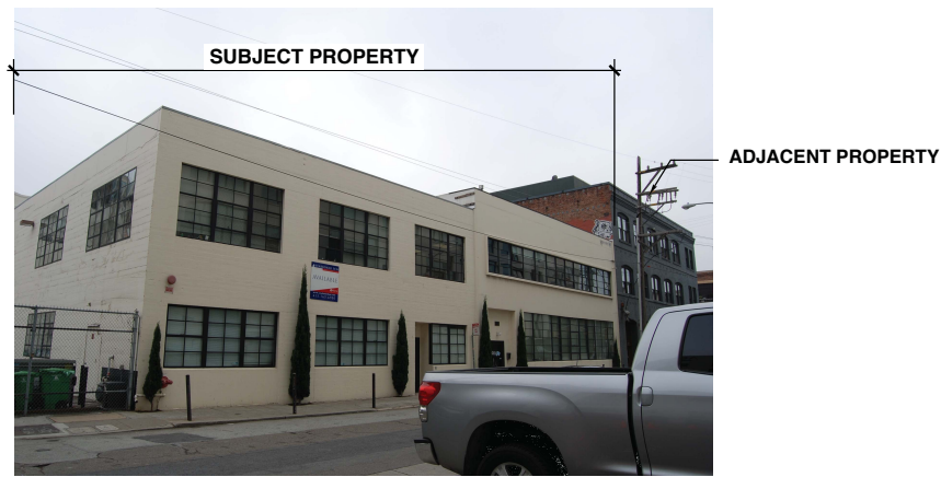
2) FEDERAL STREET: VIEW LOOKING WEST
