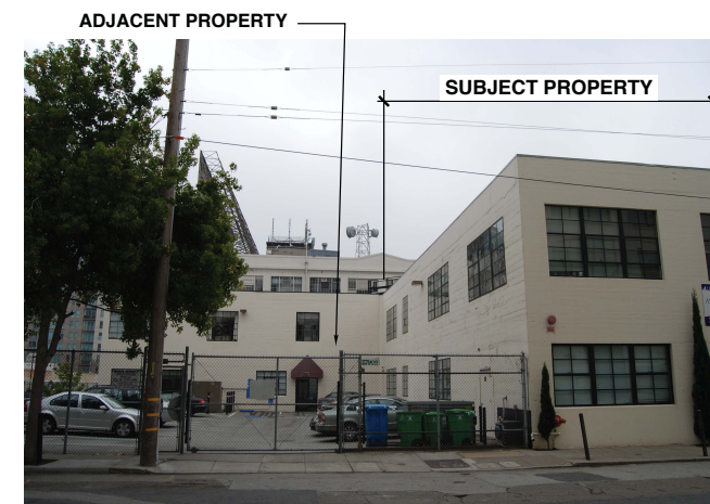
3) FEDERAL STREET: VIEW LOOKING SOUTH EAST (ADJACENT PROPERTY)
