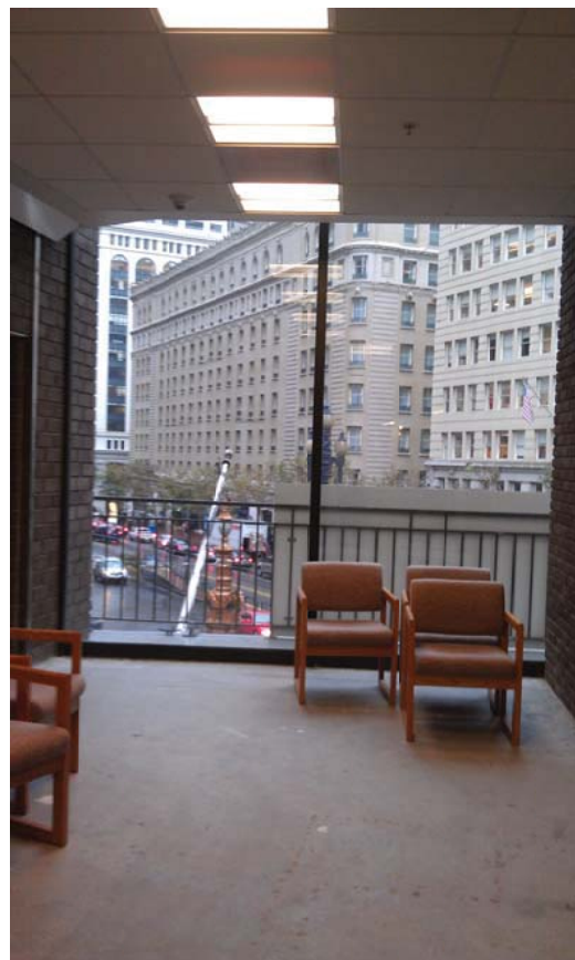
2nd Floor Lobby – Existing Interior Condition
