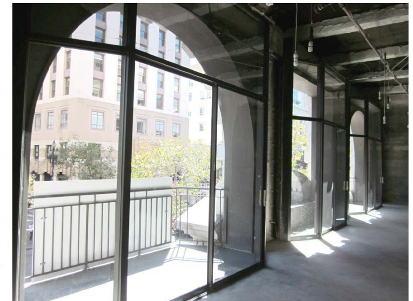
Existing 2nd Floor Windows
