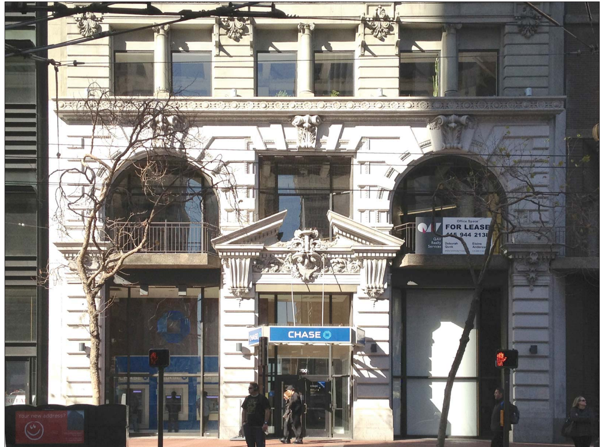
Existing Exterior Elevation Market Street
