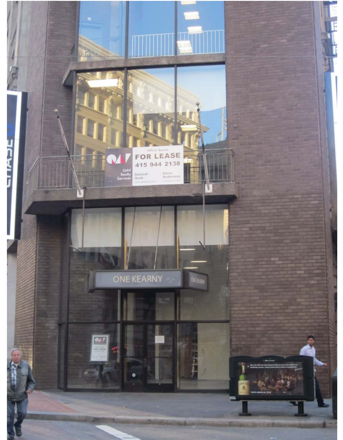
Lobby – Existing Exterior
