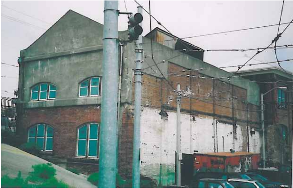
16. Powerhouse view of the south and east walls
