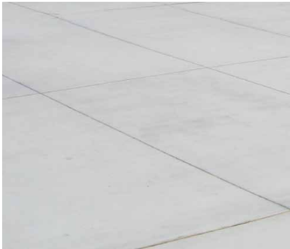
Saw-Cut Natural Concrete
