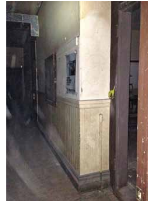
40. Office Building Second Floor north wing hallway wainscot
