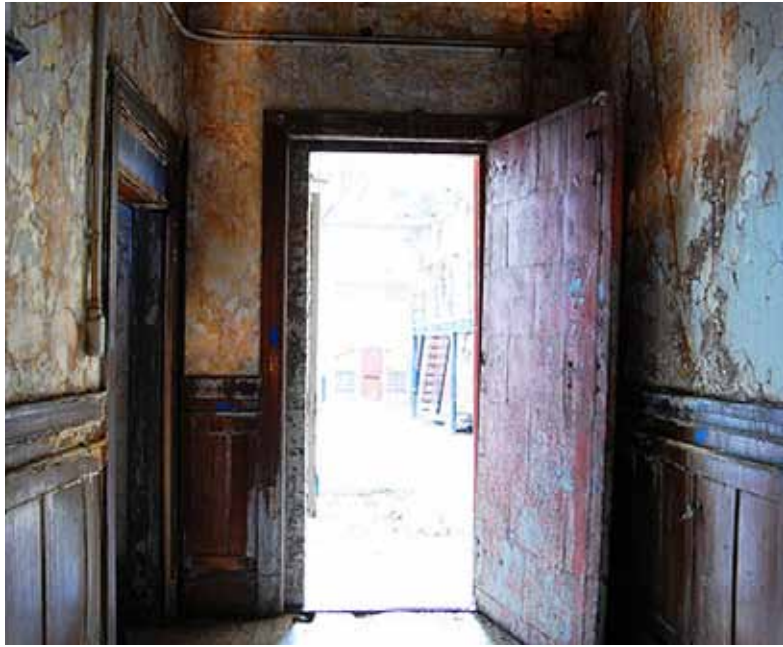
29. Office Building south wing view of door to Powerhouse
