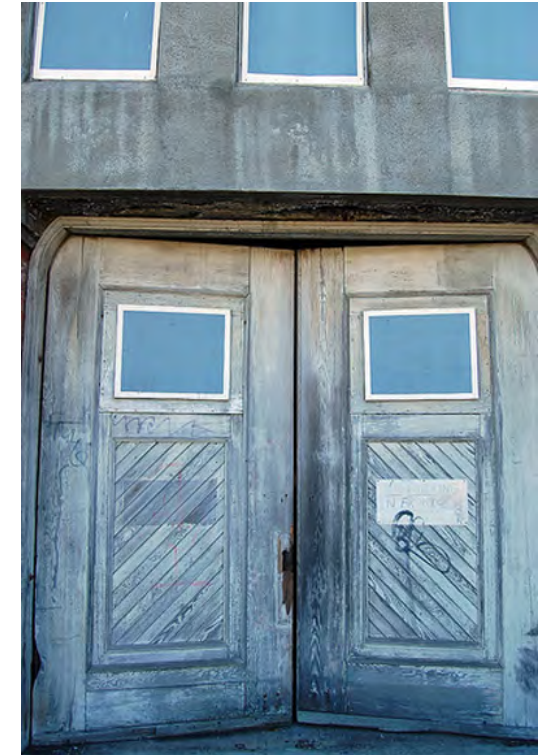
11. Powerhouse north entrance
