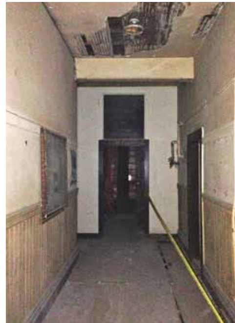
39. Office Building Second Floor north wing hallway
