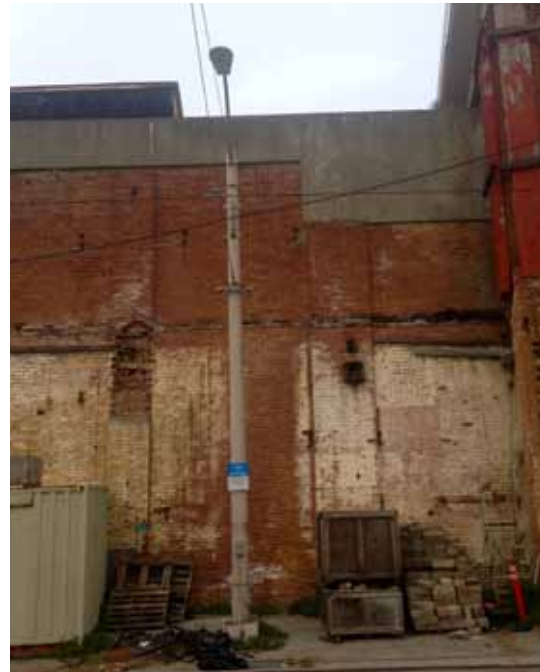
20. Powerhouse east elevation view of bricked in door opening
