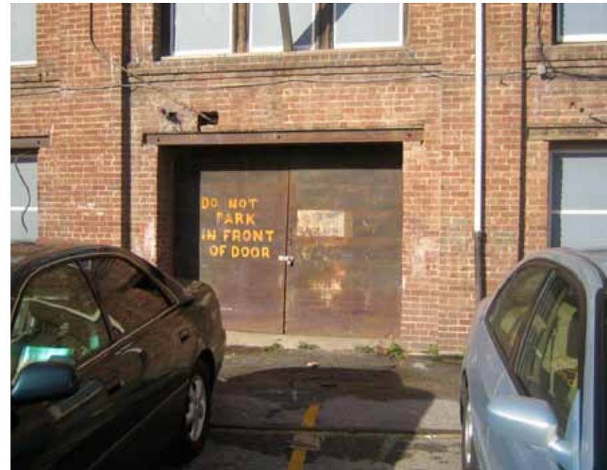
21. Office Building east elevation service doors to basement
