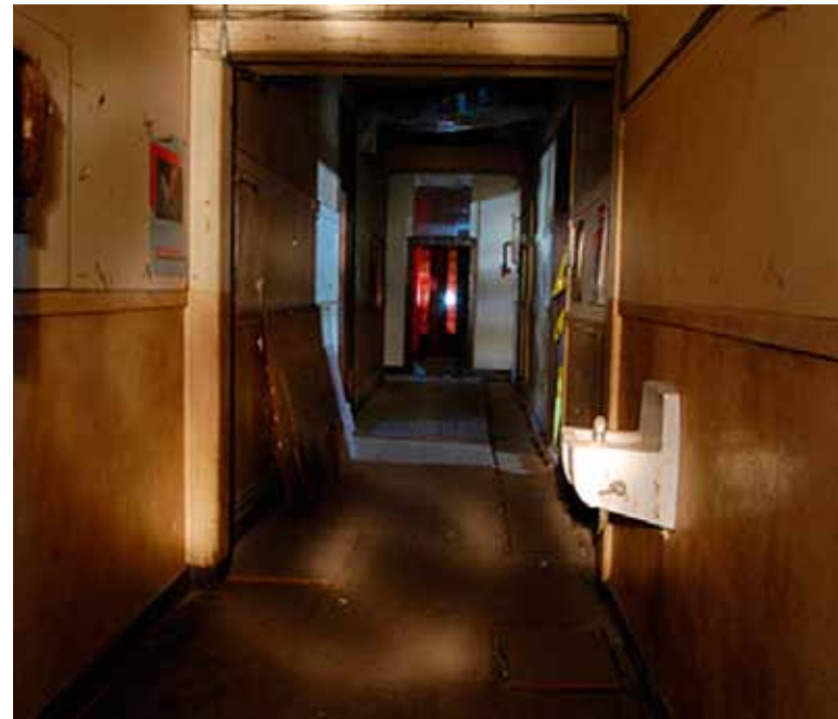
38. Office Building Second Floor south wing hallway infill looking north
