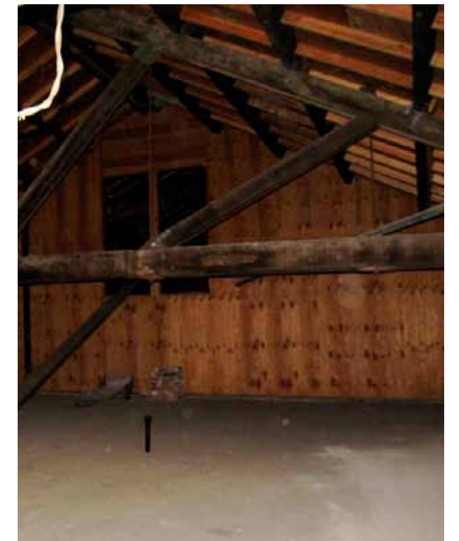
44. Office Building north wing view of attic
