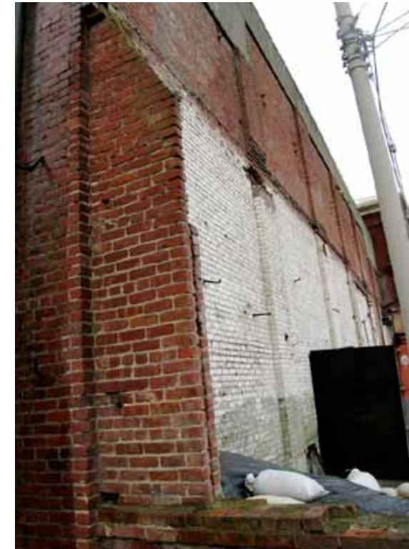
18. Powerhouse southeast corner wall fragment
