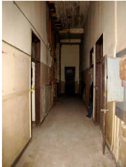
37. Office Building Second Floor south wing hallway infill looking south
