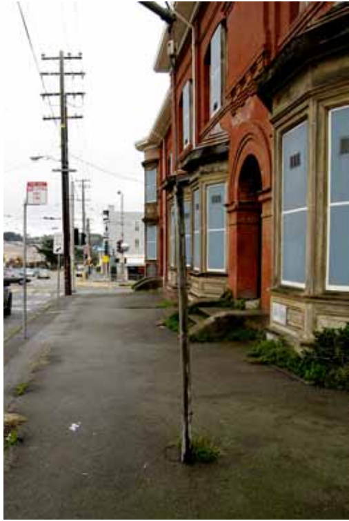
7. Office Building sidewalk and entrances
