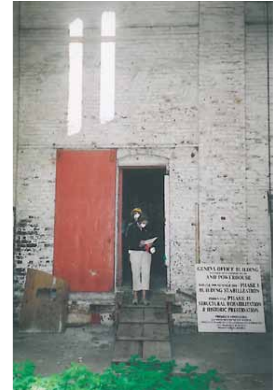
28. Powerhouse interior view of door opening to Office Building
