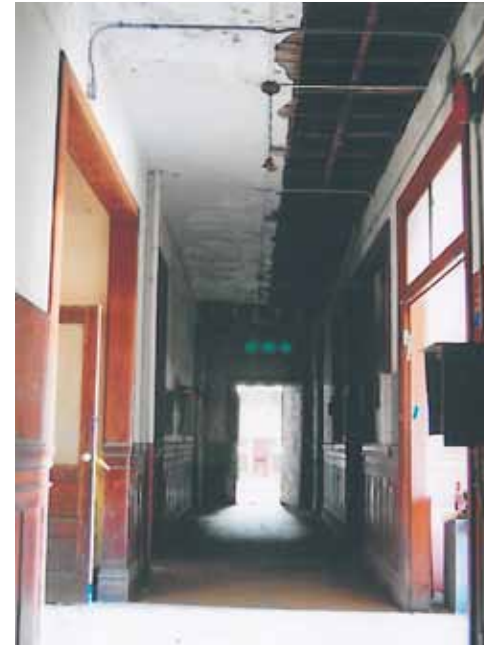
31. Office Building south wing view of corridor at entry hall
