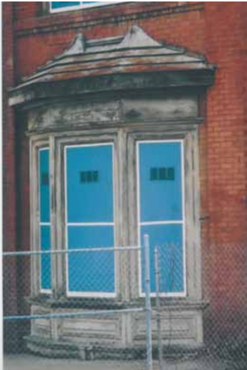
12. Office Building west elevation view of typical bay
