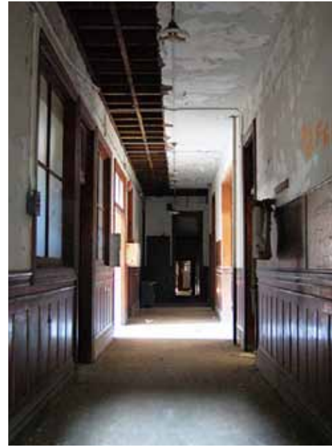
30. Office Building south wing corridor looking north
