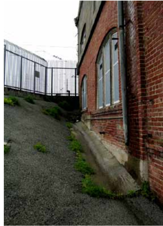
17. Powerhouse view of sloped embankment at south elevation.
