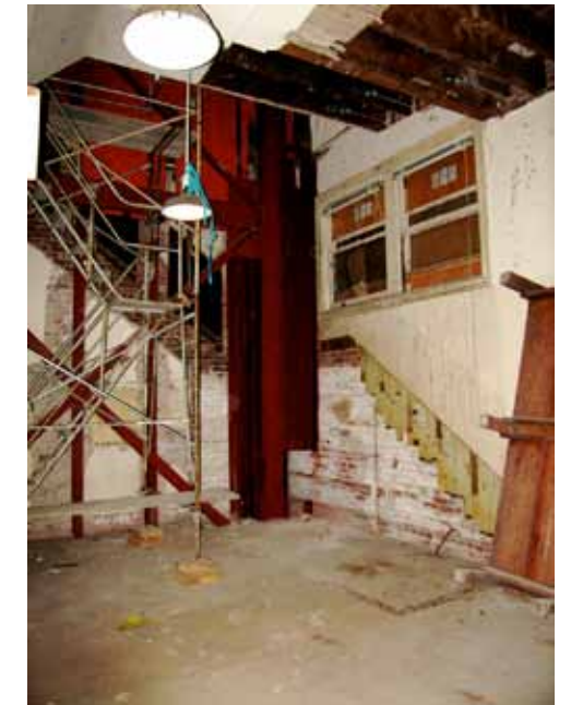
36. Office Building north wing view of northeast corner
