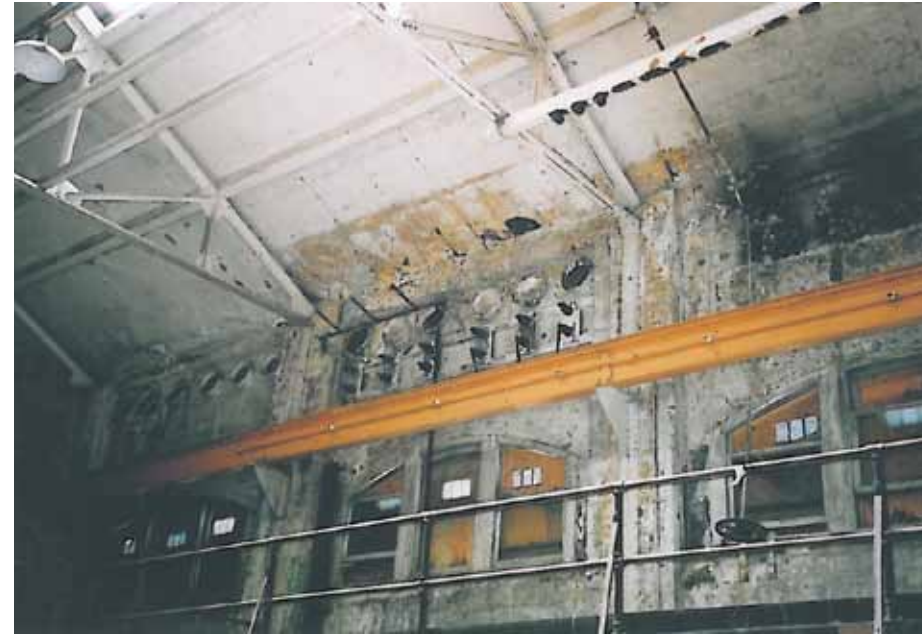
24. Powerhouse interior view of upper west wall
