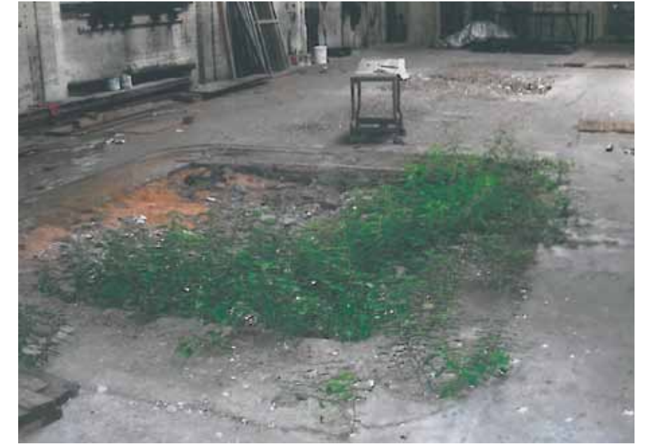
25. Powerhouse interior view of former turbine location
