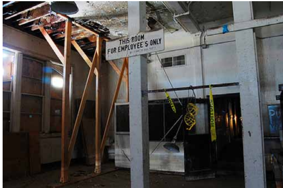
34. Office Building north wing view looking southeast
