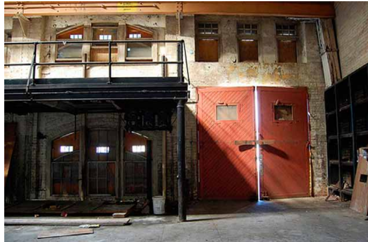
27. Powerhouse interior view of west mezzanine and entry doors
