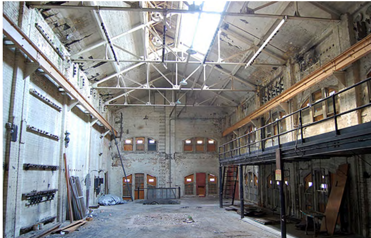
26. Powerhouse interior view looking south
