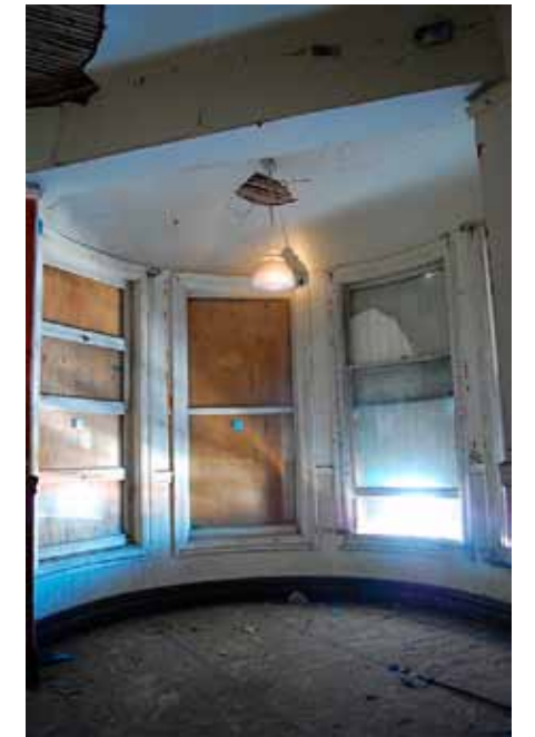
41. Office Building Second Floor north wing view of turret
