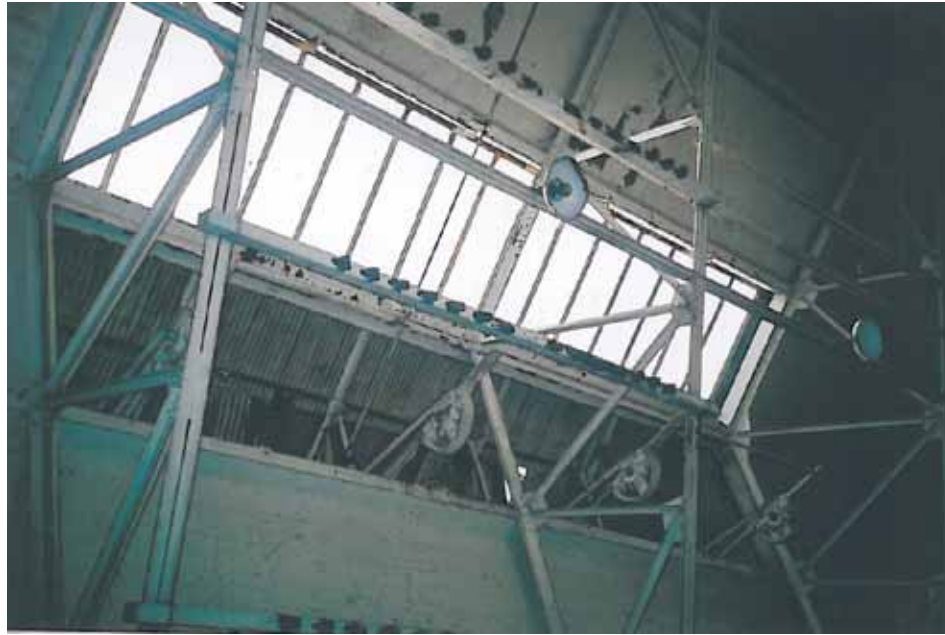
23. Powerhouse interior view of skylight
