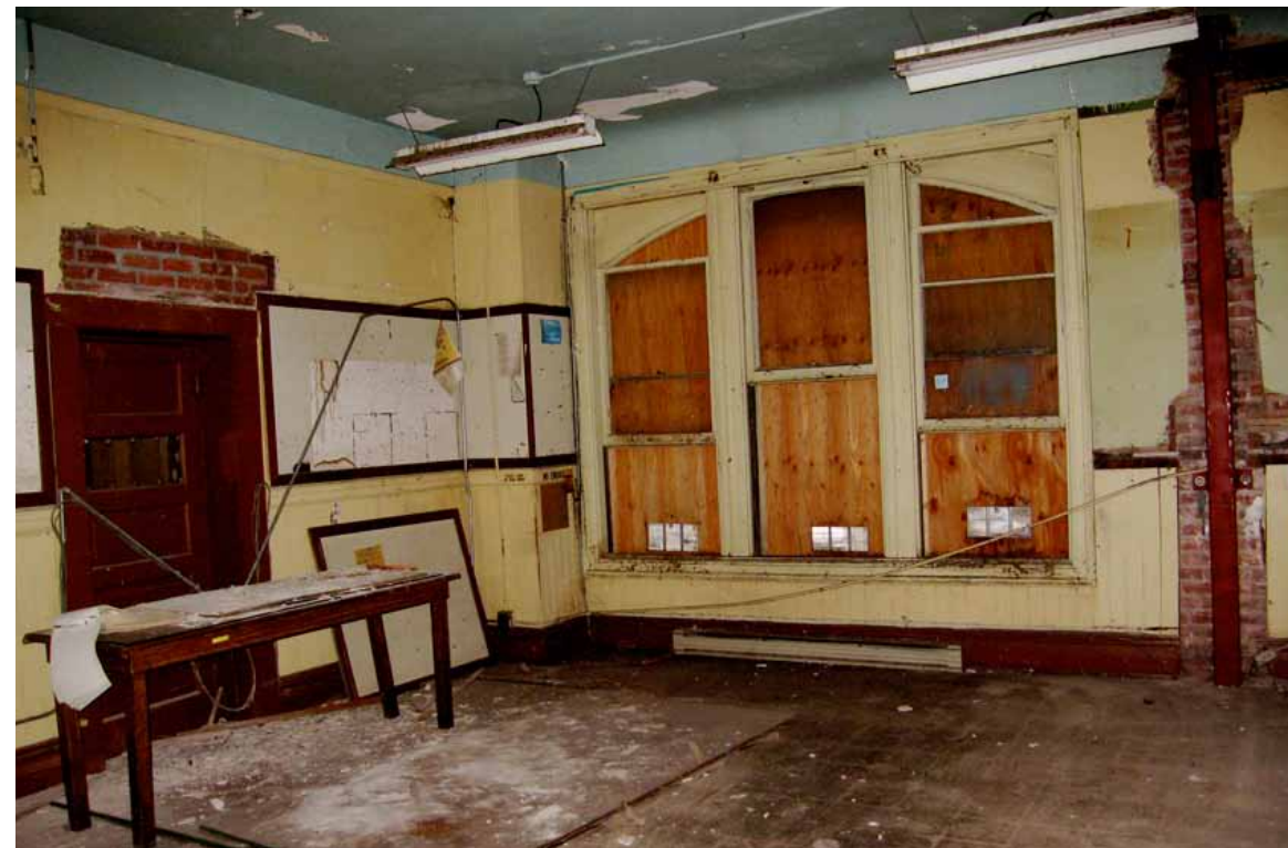
43. Office Building Second Floor north wing room
