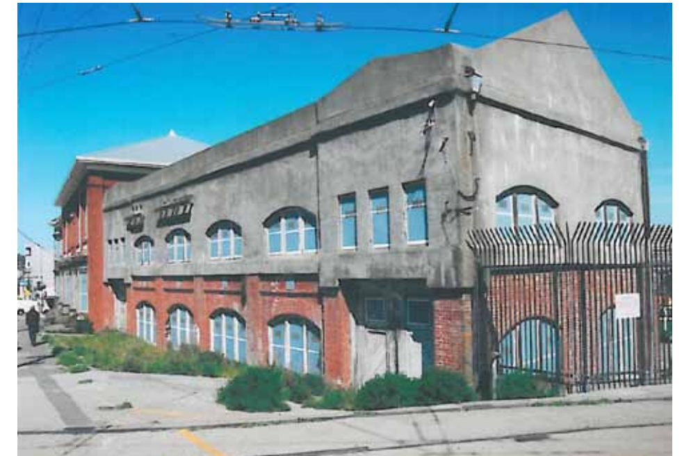
6. Powerhouse view of west and south walls
