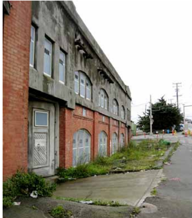
8. Powerhouse sidewalk and sloped entrances
