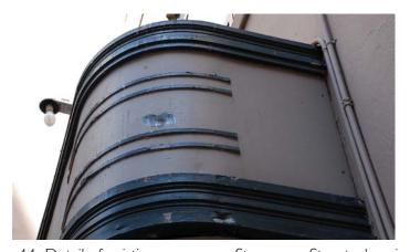
44. Detail of existing canopy on Stevenson Street, showing deterioration of the sheet metal face
