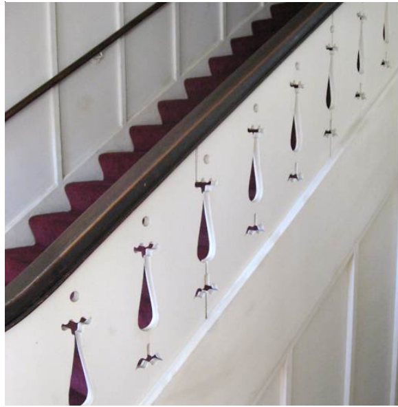
Detail of the staircase.
