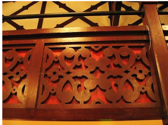
Detail of balcony fretwork
