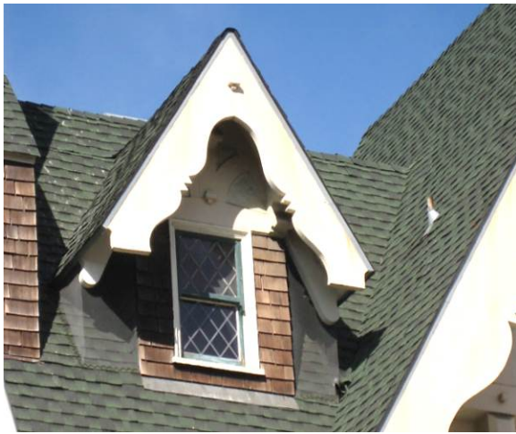
Gable dormer at the west end of the roof.
