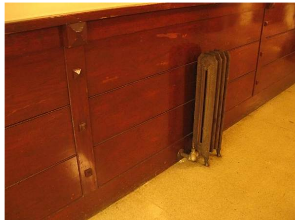
Detail of wainscot in the Valhalla room
