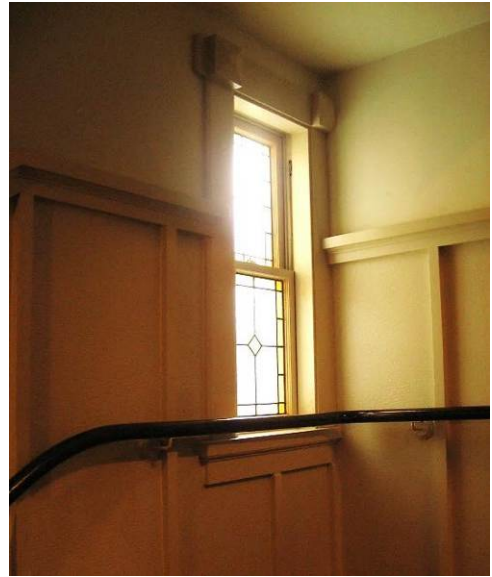
Detail of leaded glass window at the quarter-turn landing of the staircase.
