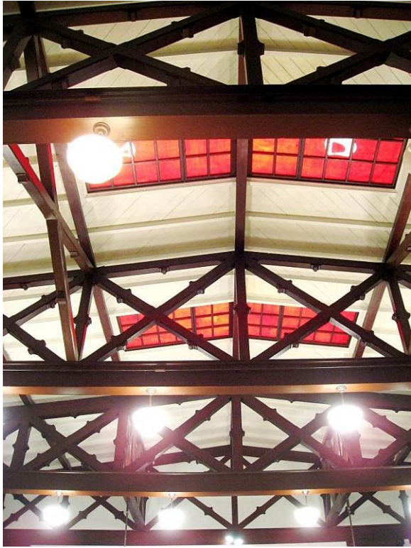
Detail of skylights
