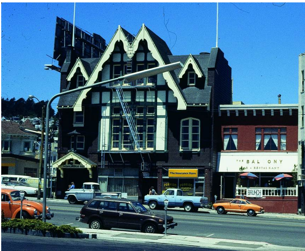
The Swedish American Hall in June, 1978. One of the few historic exterior photos of the building. Note the altered storefronts and the loss of the stepped parapets at the east and west ends of the roof. (Max Kirkeberg Collection, San Francisco State University)
