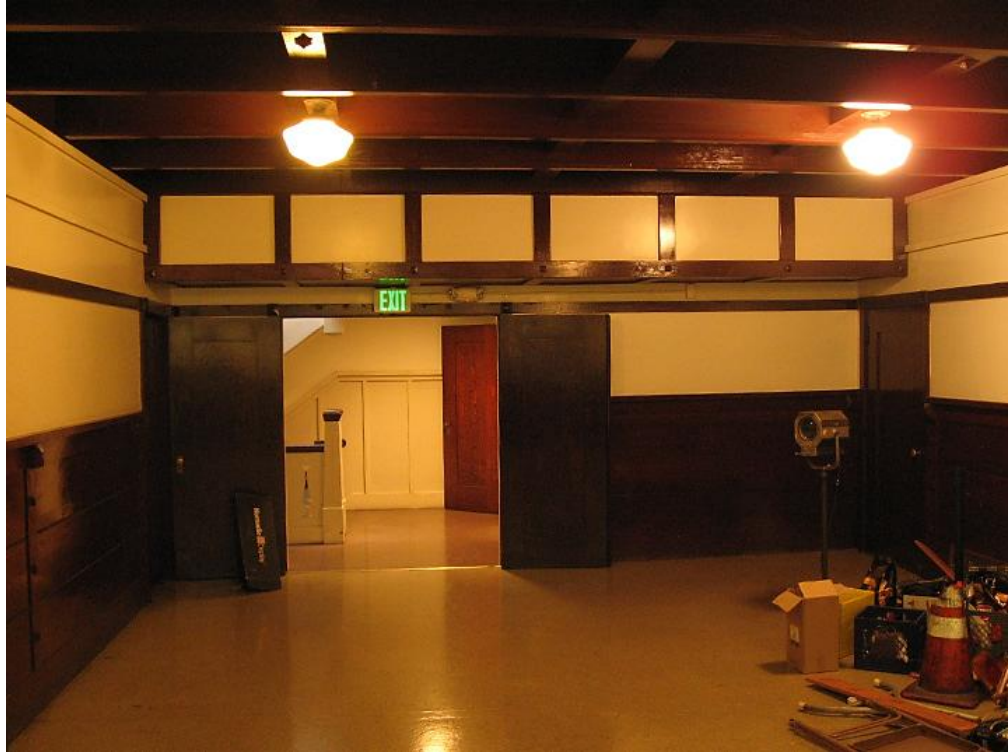
View west in the Valhalla room toward the mezzanine level stair landing.
