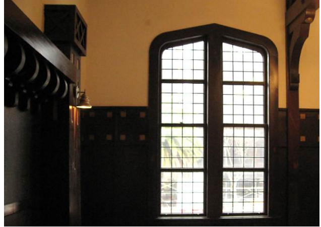
Detail of arched window near the southeast corner of the room
