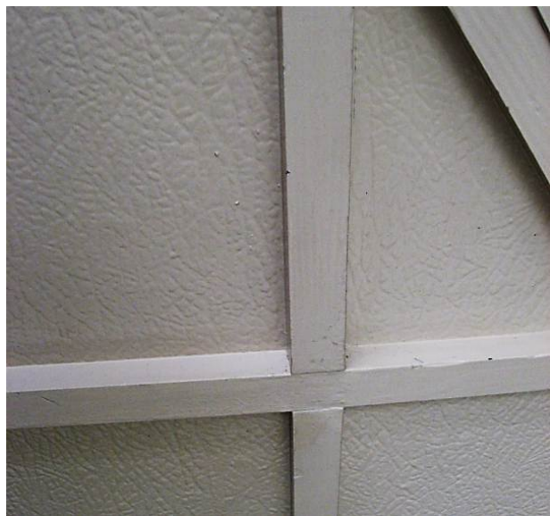
Detail of the leather paper wall cladding
