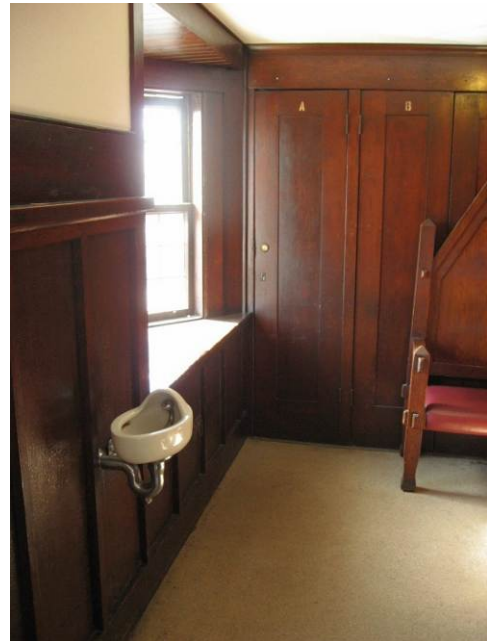
Detail of ante room with pointed bay window at left.
