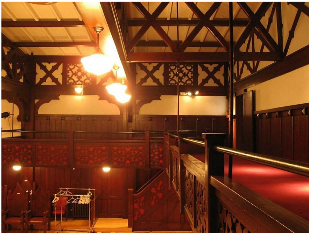
*View east along the balcony. Note the metal bars which help suspend the balcony above the floor.*
