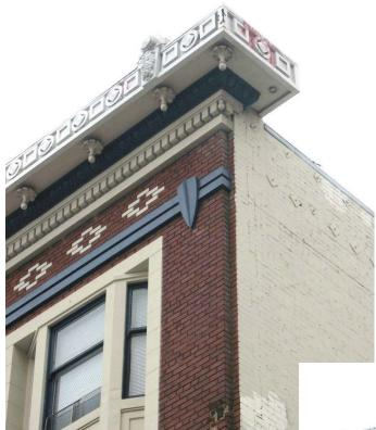
Figure 3 - 150 Franklin entablature detail
