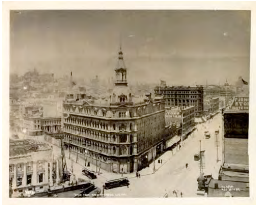
Figure 4: The Hibernia Bank building under construction at lower left, ca. 1891
