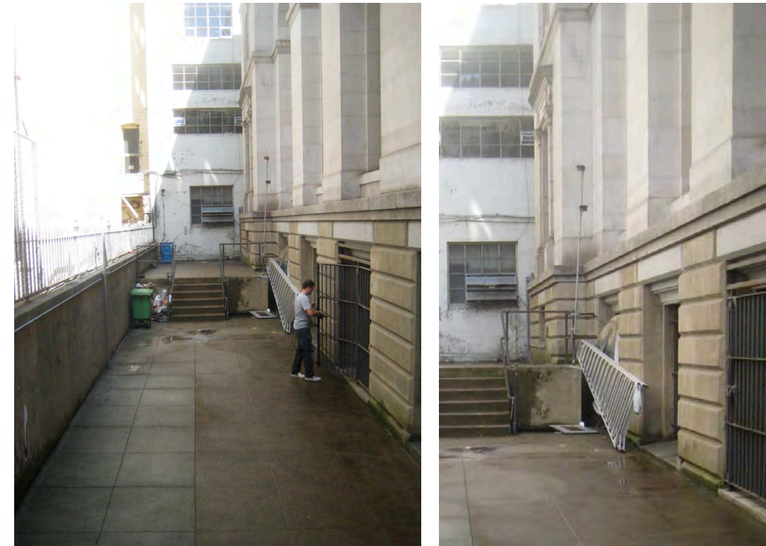
Figure 15: The west alley light well is sunken, but not to the basement floor level. The gate at the center is the access door to the basement and there are 6 steps down to the basement floor level (right). The material below the water table course is stucco over brick except for the lintels, which are granite (left).
