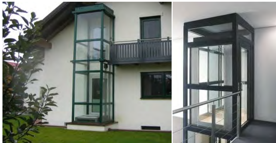
Figure 16: Examples of the proposed HC-lift. These are for illustration only. Actual lift will have inboard steel with structural glass exterior. Steel frame will be painted to reference grey granite of the building. The final design will be reviewed by the planner prior to construction.
