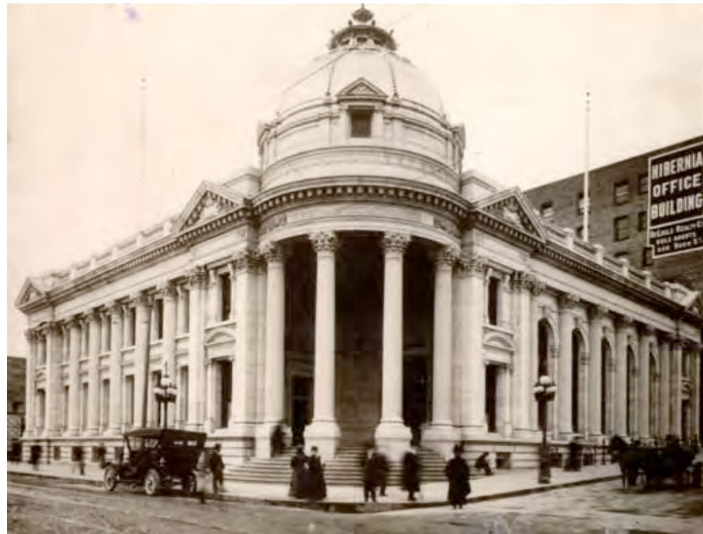
Figure 8: The Hibernia Bank Building, circa 1930
