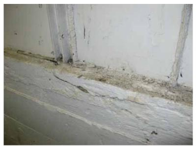
Figure 11: Concrete spalling due to steel "T" corrosion (Brannan St.).
