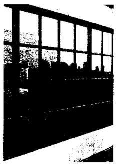
Figure 7. Despite the difficulty encountered with proper glass sizing and spacer alignment in the sealed insulating glass, the end result is an innovative window that is both aesthetically pleasing and closely matches the historic appearance of the original steel design. The slight encroachment of the bronze spacer onto the visible glass area is not readily detectable from general view. Photo: Charles Fisher
