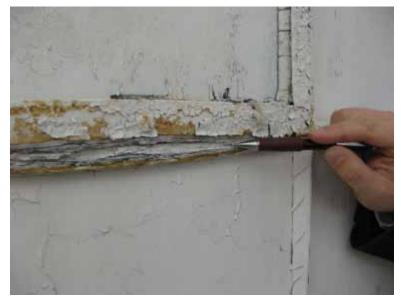
Figure 8; Corrosion leading to deformation of the steel window frame (Eight St.)
