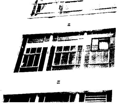
Figure 1. Many of the original Lupton windows incorporated a pair of stacked ventilators that projected outward. The vents were centrally located within a multi-light frame each of which was set either individually or in groups of two or three. Photo: Bruner/Cott & Assoc., Inc.
