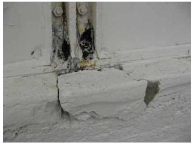
Figure 10: Concrete spalling at structural steel "T" (Eight St.).
