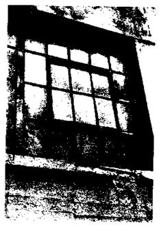
Figure 2. Due to lack of maintenance, severe rusting of the steel frames had occurred, which contributed to the spalling of sections of the concrete sills, jamhs, and spandrels. Photo: Charles Fisher
