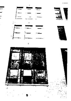
Figure 4. Among the retained and repaired original windows were these large units on the second floor level. Photo: Bruner/Cott & Assoc., Inc.
