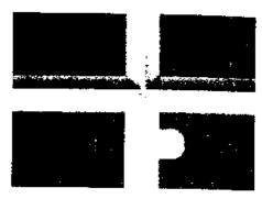
Figure 4. The vertical muntins had mitre joints where they intersected the horizontal muntins and were secured through a combined use of epoxy glue and spot welding. Photo: Charles Fisher
