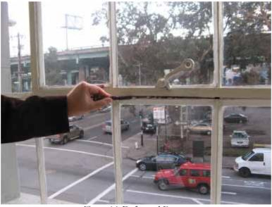
Figure 16: Deformed Frame.
