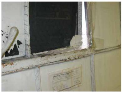
Figure 9: Warped ventilator no longer closes properly (Brannan St.)
