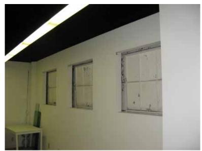
Figure 6: Interior finishes covering window except operable vents (Brannan St.)
