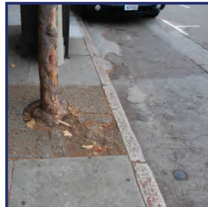
6" granite curb at McAllister St
