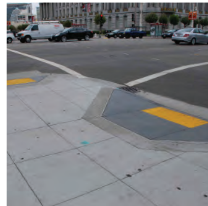
Curb ramp at McAllister St and Van Ness Ave
