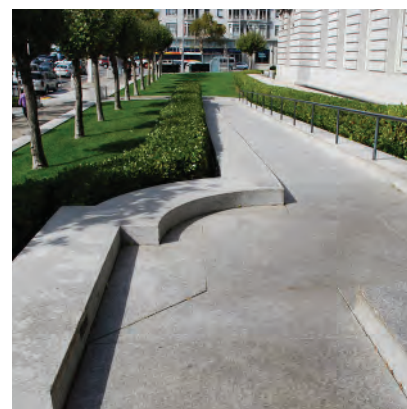
Accessible granite ramp to City Hall's west entrance at Van Ness Ave
