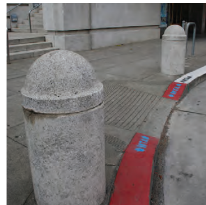
Concrete bollards with domed tops along Grove St
