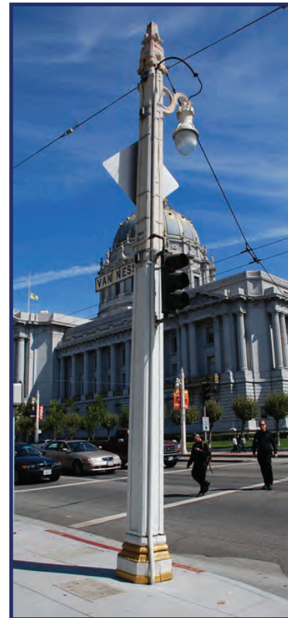
Van Ness trolley pole with single pendant
