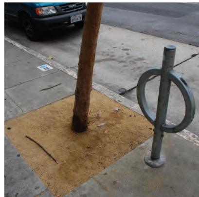
Square tree well with DG fill and ring and post style bike rack along Van Ness Ave
