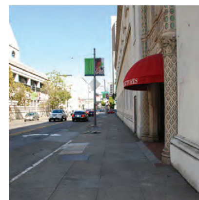
Concrete sidewalk paving pattern along Hayes St
