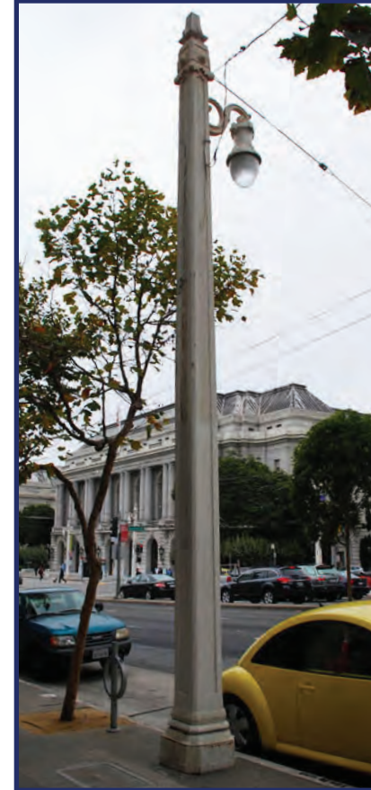
Van Ness trolley pole with single pendant
