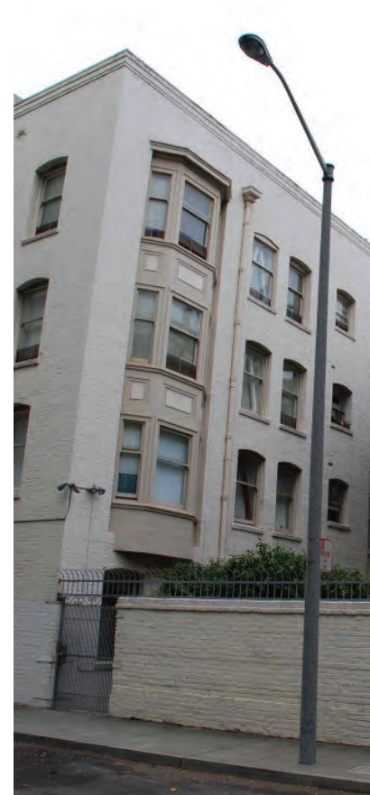
Single cobra street light on Redwood St
