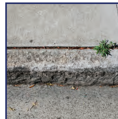
6" granite curb along Fell St
