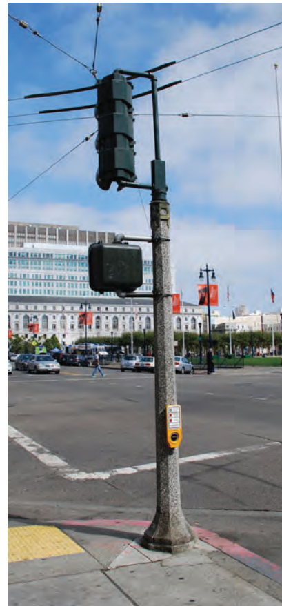
Modified aggregate concrete post with traffic signal
