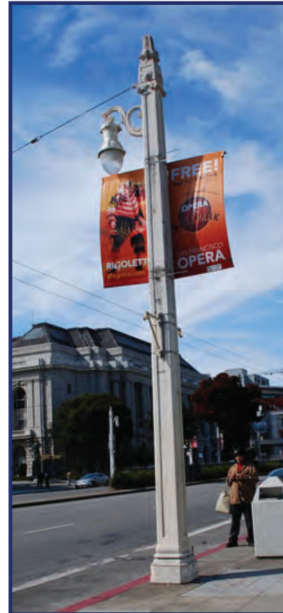
Van Ness trolley pole with single pendant
