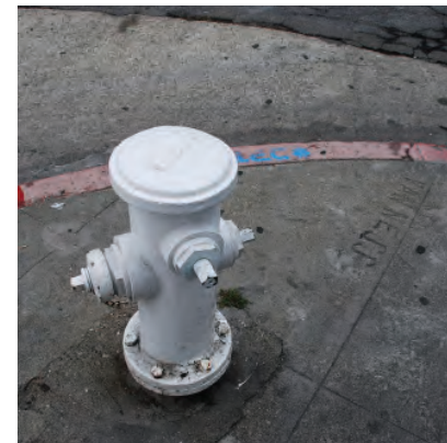
Low pressure hydrant at Redwood St
