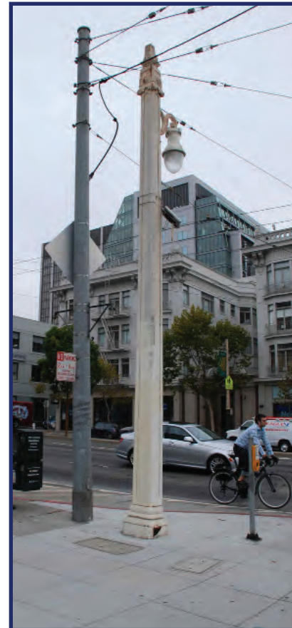
Van Ness trolley pole with single pendant
