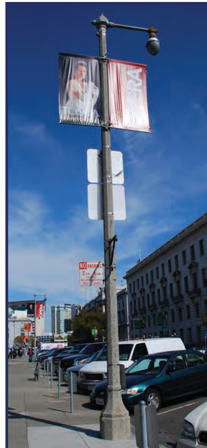
Aggregate concrete streetlight post with right angle pendant on Grove St
