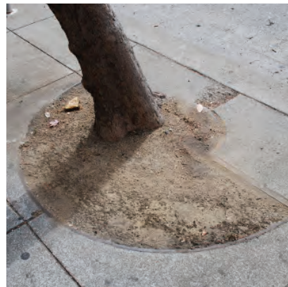
Tree well along Hayes St - semicircle, no grate, filled with decomposed granite
