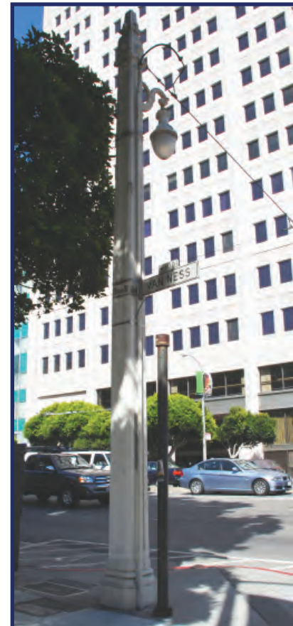
Van Ness trolley pole with single pendant
