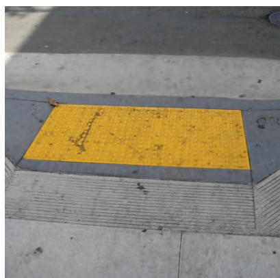
Accessible ramp with truncated domes
