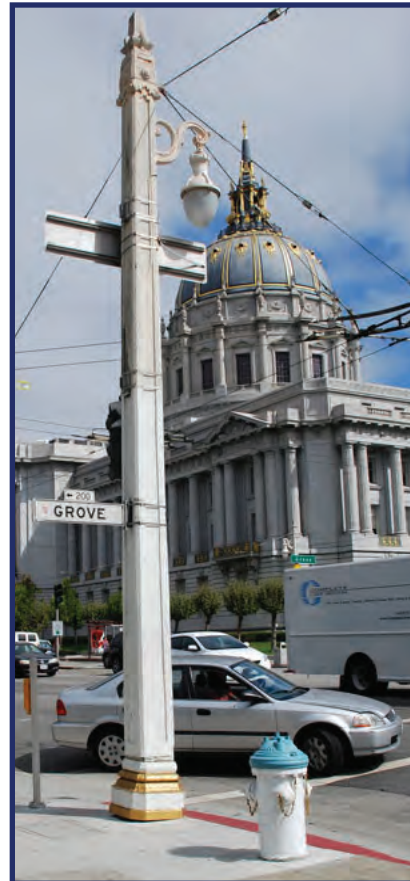
Van Ness trolley pole with single pendant and high pressure auxiliary water supply hydrant
