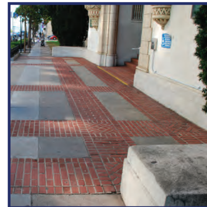
Brick paving pattern along Van Ness Ave
