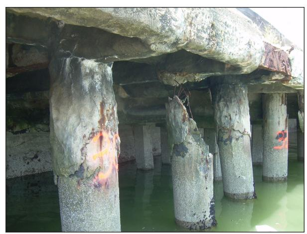
View of Deteriorated Bulkhead Wharf Substructure Piles
