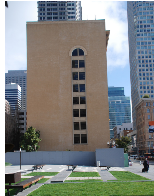
View of Aronson Building from west, Jessie Square in foreground. (Page & Turnbull)
