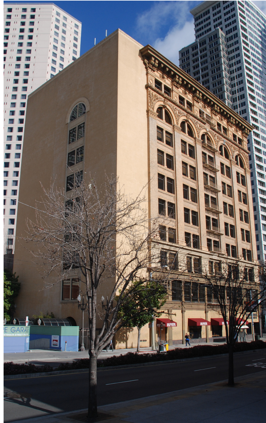
View of building along Mission Street. (Page & Turnbull)
