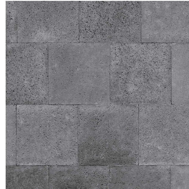
STONE @ ENTRY WALL recinto volcanic rock
