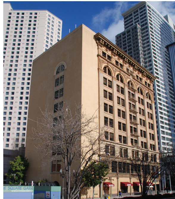
View of Aronson Building from southwest, Westin Hotel and UC Berkeley Extension in background. (Page & Turnbull)
