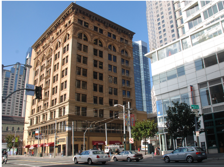
View of Aronson Building from southeast, UC Berkeley Extension in foreground. (Page & Turnbull)
