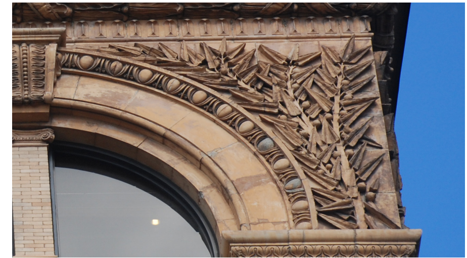
Terra cotta at the Aronson Building
