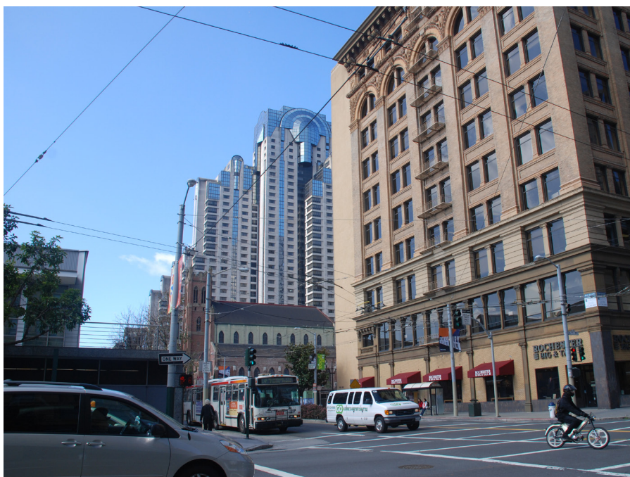
View of Aronson Building from southeast, St. Patrick's Church and Marriott Hotel in background. (Page & Turnbull)
