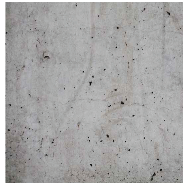
CONCRETE structural walls / columns
