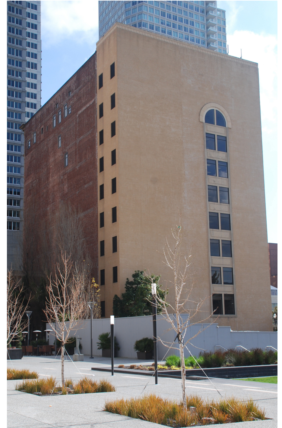
View of building from northwest. (Page & Turnbull)
