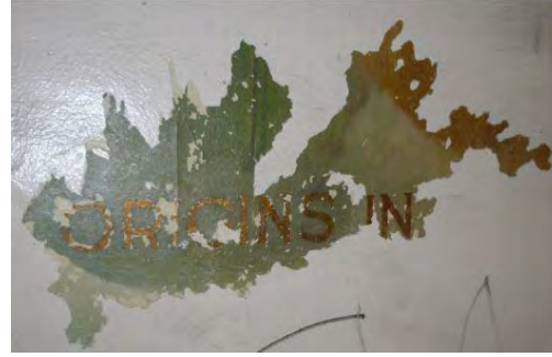
Uncovered portion of Gerrity mural. Source: EverGreene Architectural Arts memo, dated April 29, 2015.
