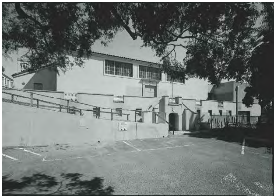
2012 Before demolition [William Porter]
