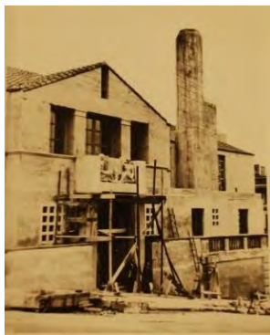
1928 Richardson Hall under construction [SFSU 039]
