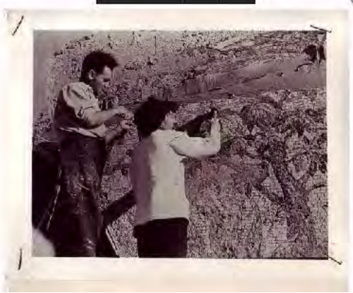
Maxine Albro and technician working to install WPA mosaic mural [National Archive and Records Administration, Neg. 8169-C]
