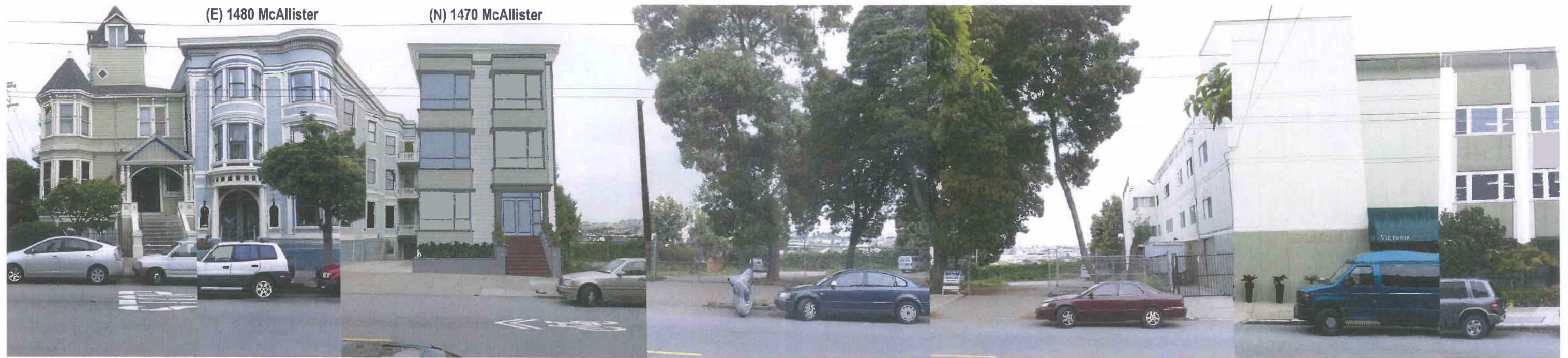
McALLISTER STREETScape SEGMENT #1
