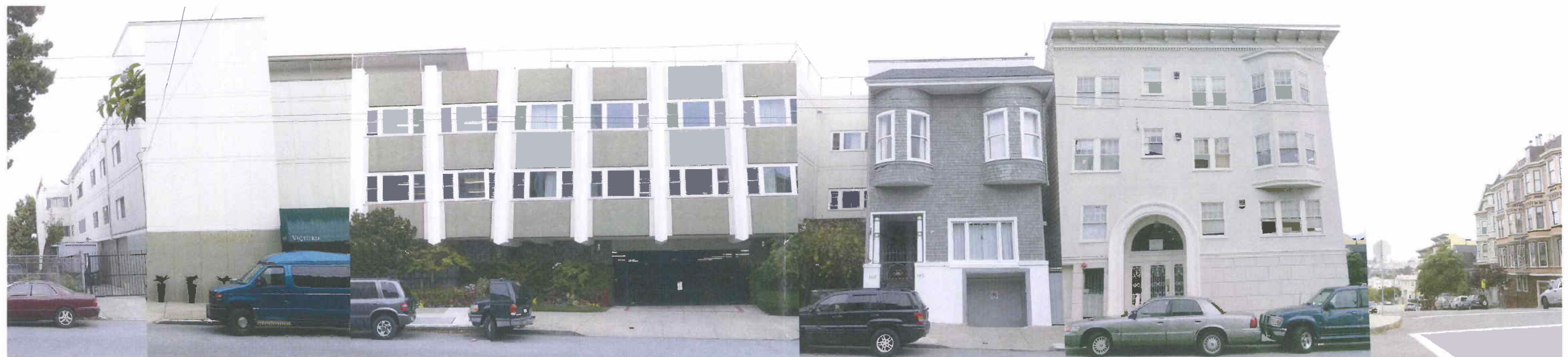
McALLISTER STREETScape SEGMENT #2
