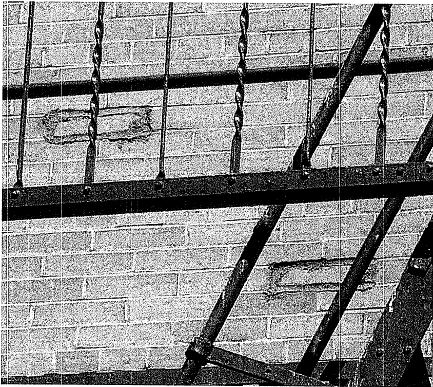
17-29 Third Street - Limited locations of mismatched mortar
