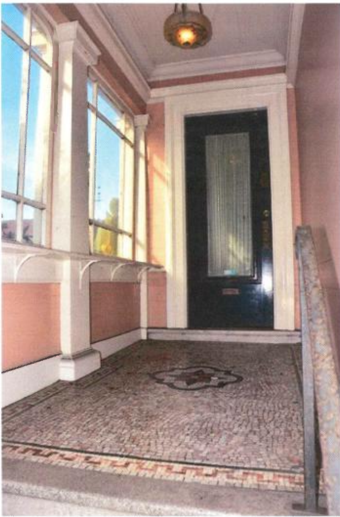
Illustration 1: 137 Clayton Front Porch & windows
