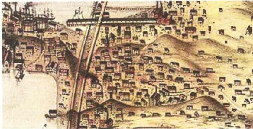
Potrero Point and Long Bridge, 1857
