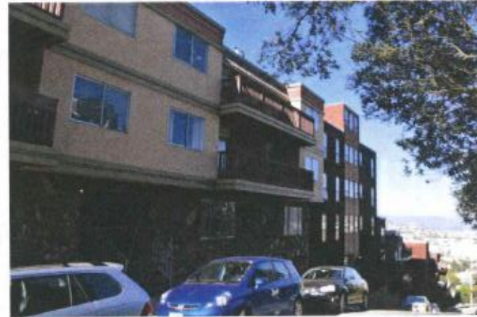
South Elevation of Adjacent Building, 550 27th Street
