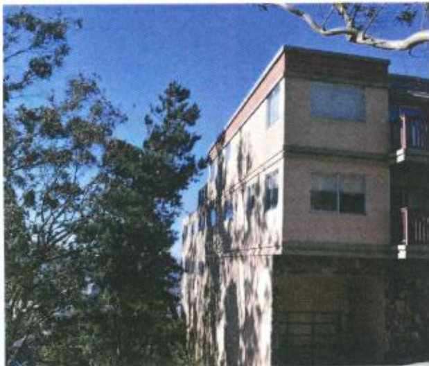
Southwest Corner of Adjacent Building, 550 27th Street
