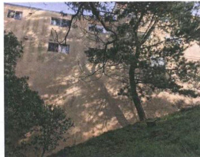
Existing Western Elevation of Adjacent Building, 550 27th Street
