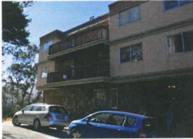
South Elevation of Adjacent Building, 550 27th Street
