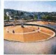
Southeast Wastewater Treatment Plant
