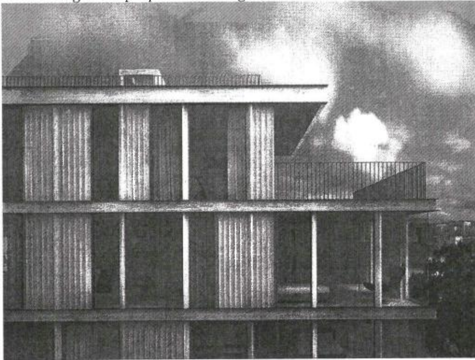
GFRC panels for new façade
