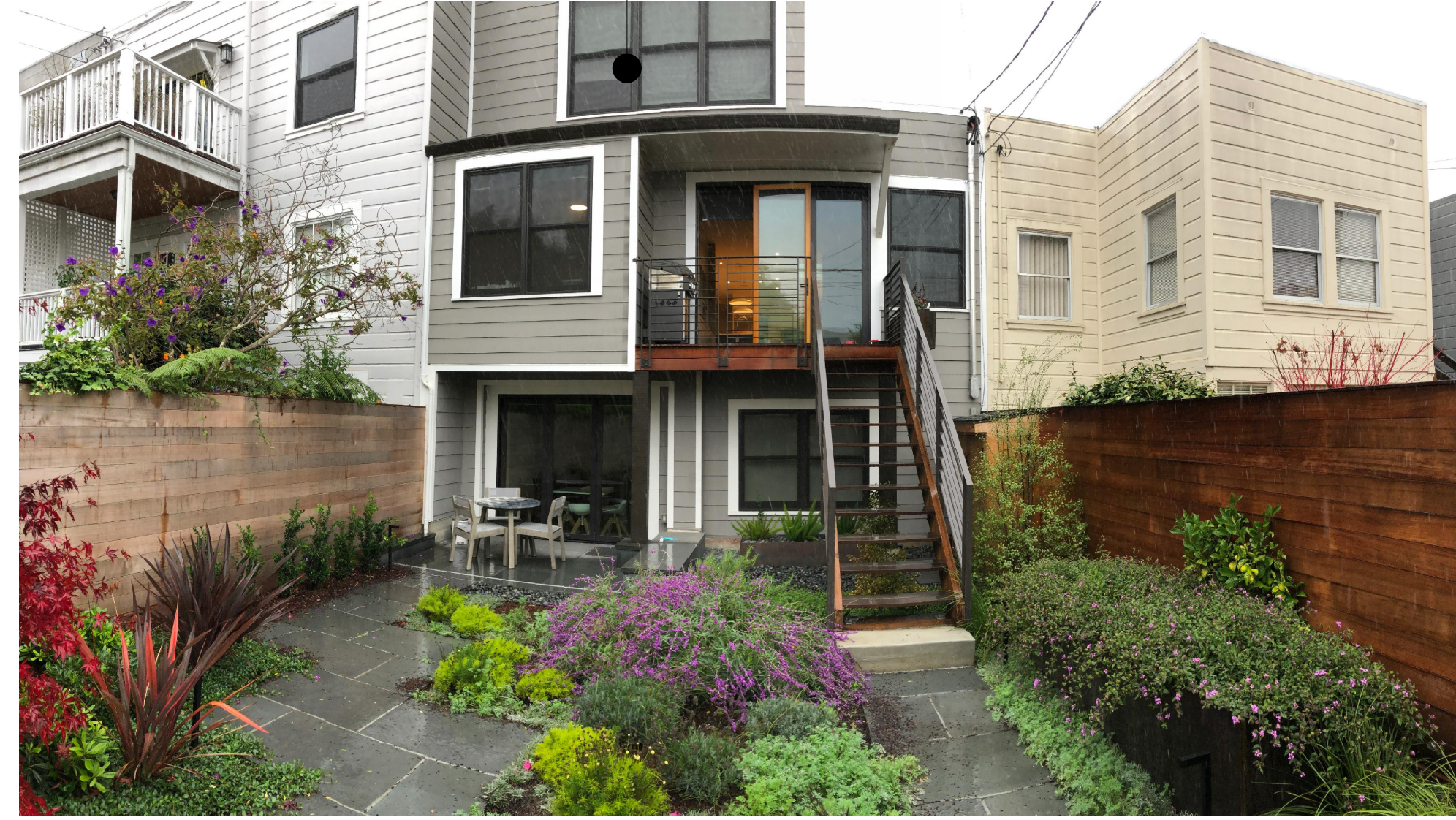
1 - REAR FACADE AND ADJACENT BUILDINGS
